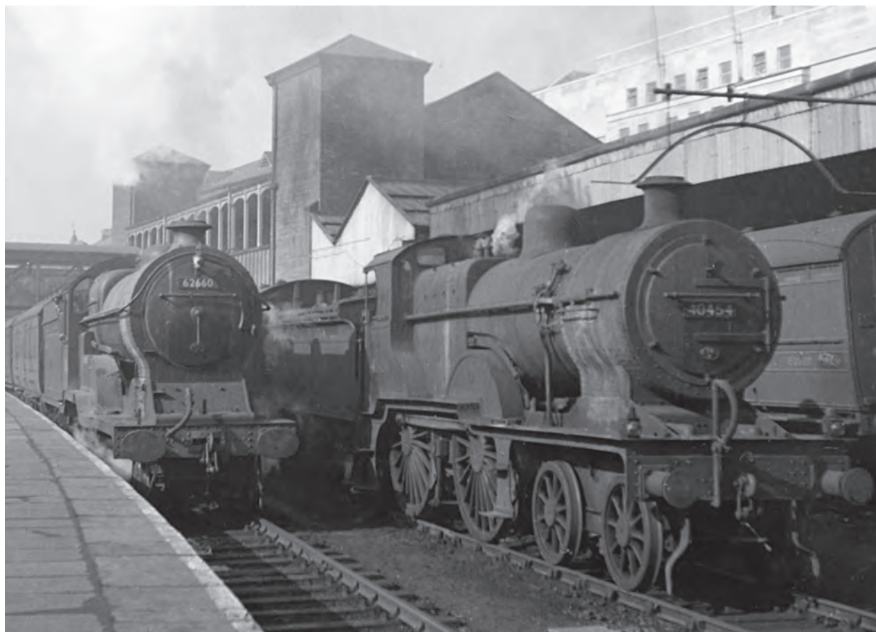
A brace of Midland locomotives, Compound 4-4-0 Class '4P' No. 41143 has been attached to Fowler 0-6-0 Class '4F' No. 44408 on an eastbound freight train passing through Nottingham Midland station on 24 December 1954. No. 41143, a product from the NBL Co. Glasgow in 1925, was withdrawn in March 1959 from Derby shed and scrapped at Crewe Works. The '4F' was built in 1927 at Derby Works, condemned from Normanton shed in October 1965 and cut up at Garnham, Harris & Elton, Chesterfield. ( M.E. Kirk/Martyn Reeve Collection )
