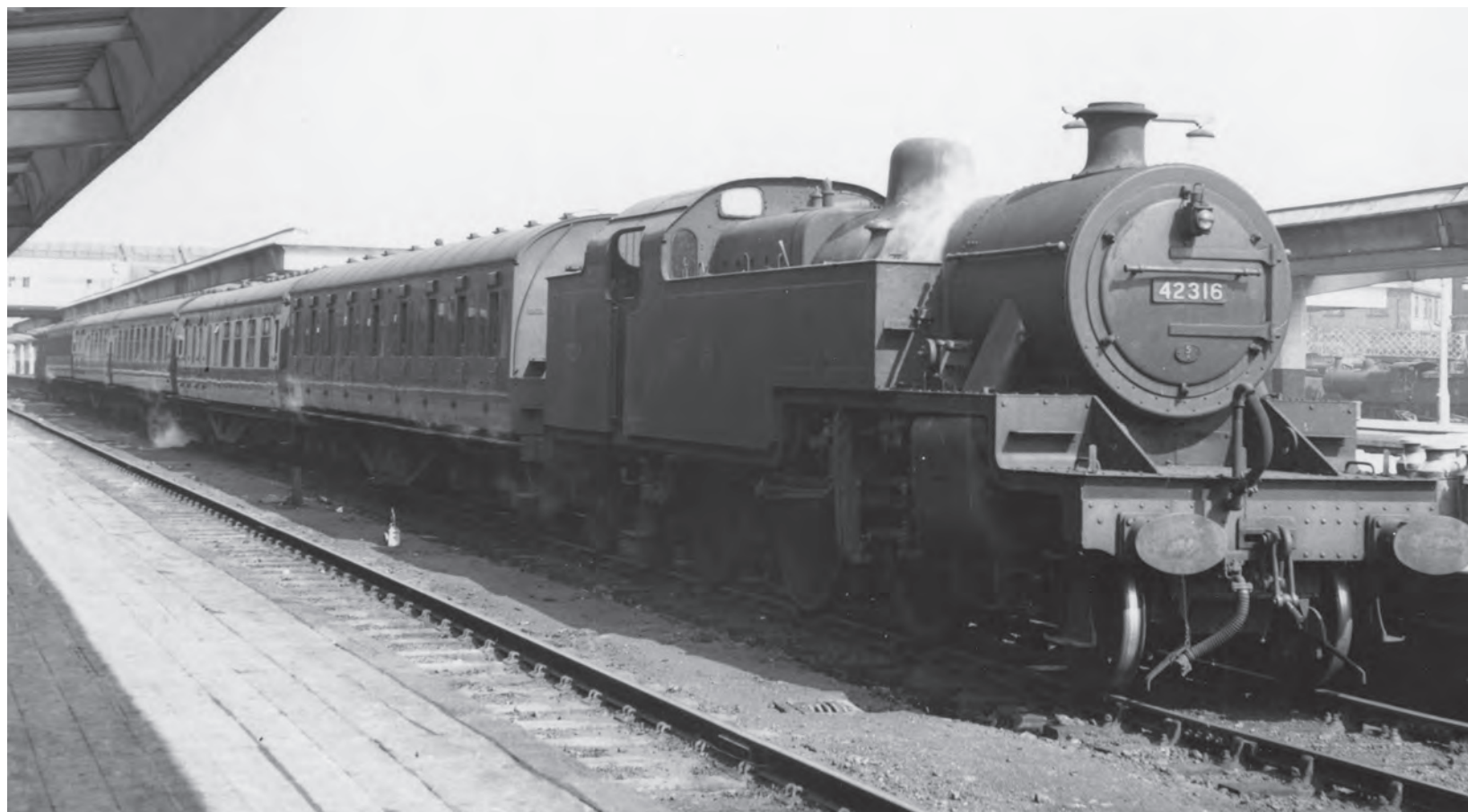
The 10.50am (Sun) Derby to Crewe stopping train waits on platform 2 on 15 April 1956 and is being worked by Fowler 2-6-4T Class '4P' No. 42316. It was built in 1928 at Derby Works and scrapped there when withdrawn from Stockport (Edgeley) shed in February 1963. (M.E. Kirk/Martyn Reeve Collection)
