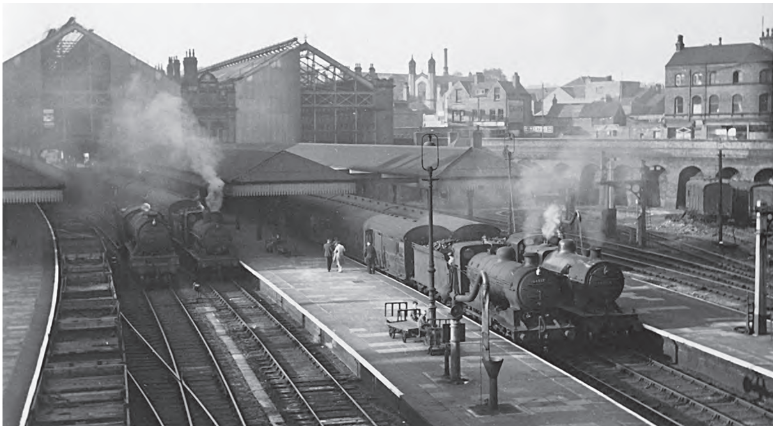
A busy evening scene at Nottingham Victoria station on 23 August 1952. Left to Right, Gresley 2-6-0 Class 'K3' 61976, built in 1936 at Darlington Works, withdrawn from Sheffield (Darnall) shed in January 1962 and cut up at Doncaster Works. Ivatt 0-6-0 'J5' No. 65487 with the 6.05pm to Basford & Bulwell via Gedling was built in 1910 at Doncaster Works and had less than a year before withdrawal from Colwick shed in June 1953. Ivatt/Gresley 0-6-0 'J6' No. 64237 waits with the 6.15pm to Grantham. This was built in 1914 at Doncaster Works and scrapped there when withdrawn in November 1959 from Hitchin shed. Johnson 4-4-0 Class '2P' No. 40534 has a while to wait before it leaves with the 6.34pm to Northampton (Castle). Built in 1899 at Derby Works, it was withdrawn from Nottingham shed in July 1959 and disposed of by T.W. Ward, Killamarsh. (M.E. Kirk/Martyn Reeve Collection)
