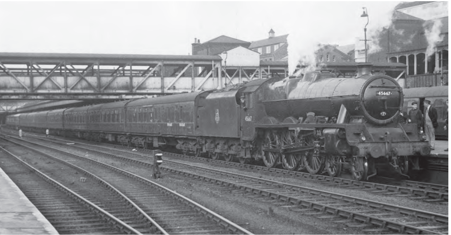
The 7.20am Bradford (Forster Square)-London (St Pancras) is arriving behind Nottingham-allocated 'Jubilee' 4-6-0 Class '6P' No. 45667 Jellicoe in August 1957. Built in 1935 at Crewe Works, Jellicoe was withdrawn from Bank Hall shed in January 1965 and cut up by Maden & McKee, Liverpool. (M.E. Kirk/Martyn Reeve Collection)
