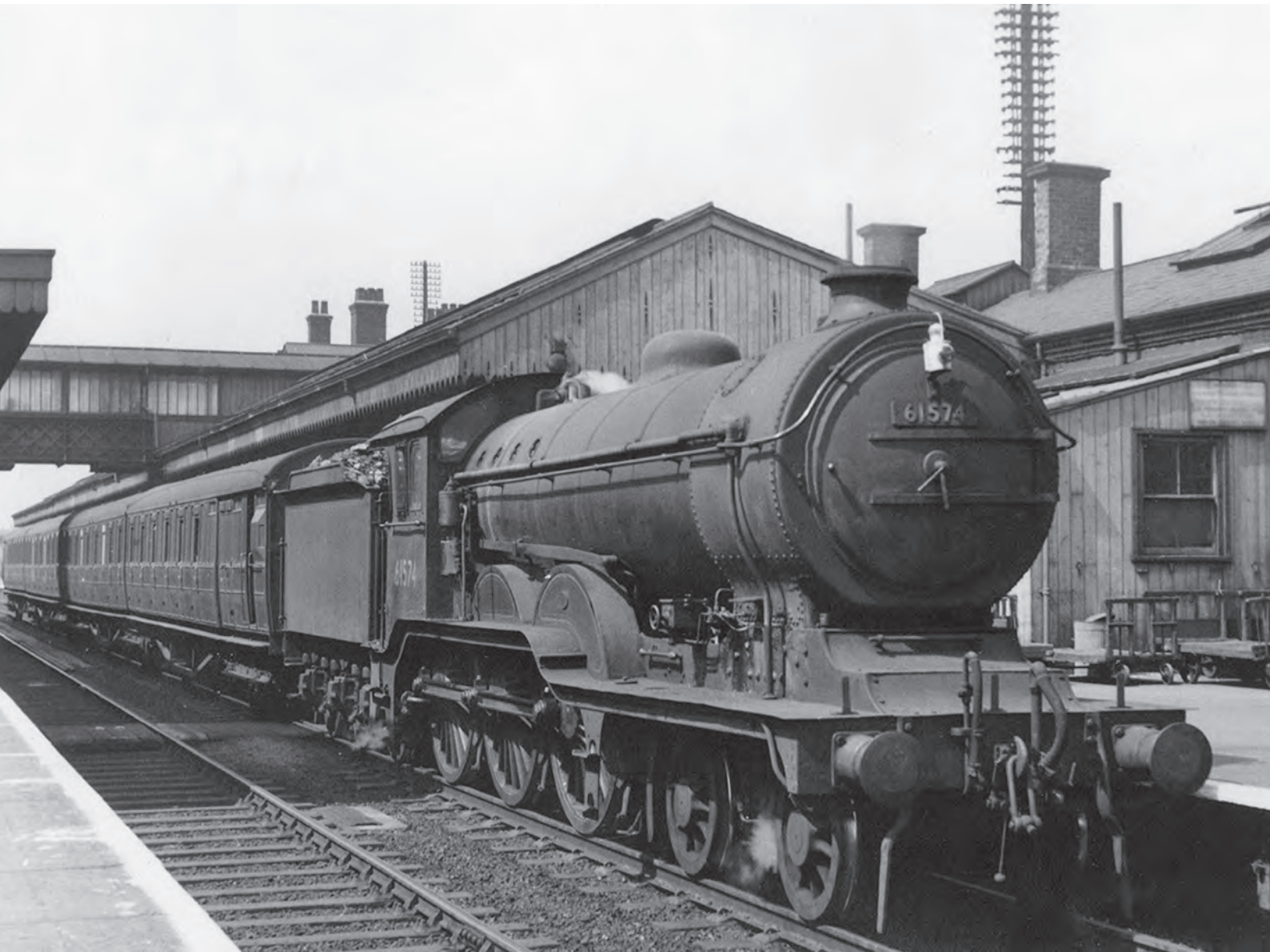
Holden designed 4-6-0 Class 'B12' No. 61574 arrives at Grantham station on 14 July 1954 with the 1.04pm service from Skegness. It was manufactured by Beyer Peacock Ltd in 1928 and withdrawn from Grantham shed in January 1957 before being broken up at Stratford Works. ( M.E. Kirk/Martyn Reeve Collection )
