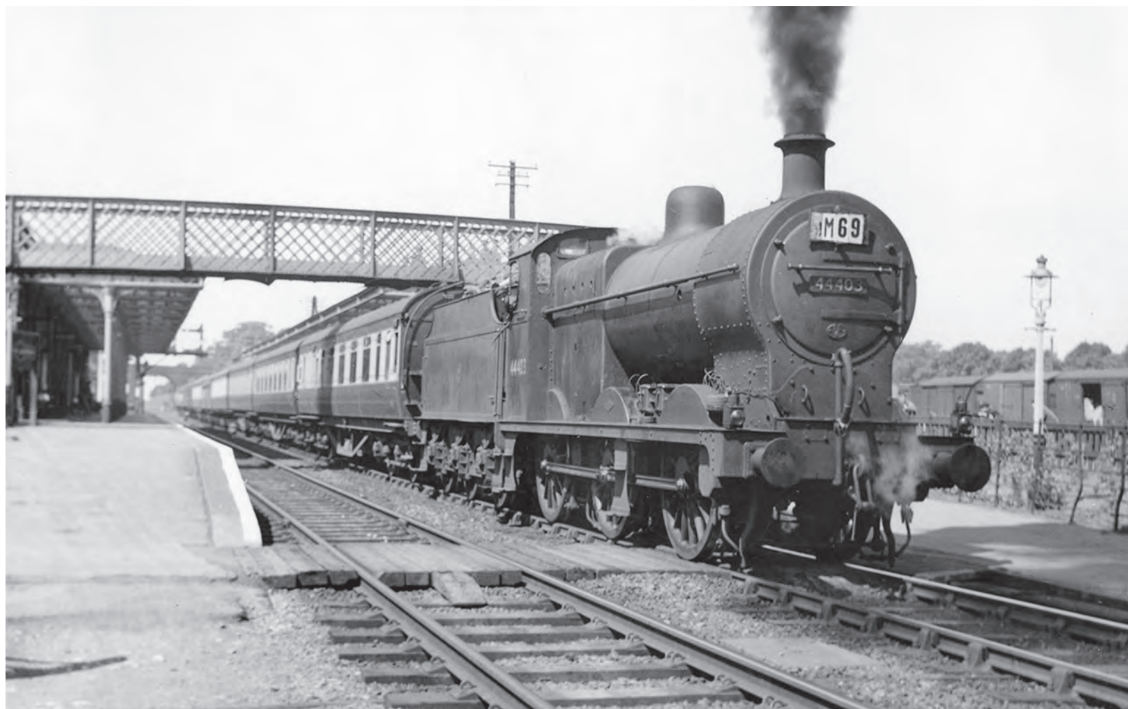
Fowler 0-6-0 Class '4F' No. 44403 is waiting to leave Melton Mowbray (Town) on 19 July 1952 with the 9.05am (SO) Kings Norton-Yarmouth (Beach) and Lowestoft (Central) train. Manufactured in 1927 by North British Locomotive Co. Glasgow, this locomotive was withdrawn from Coalville shed in June 1964 and broken up at Cashmore's, Great Bridge. (M.E. Kirk/Martyn Reeve Collection)
