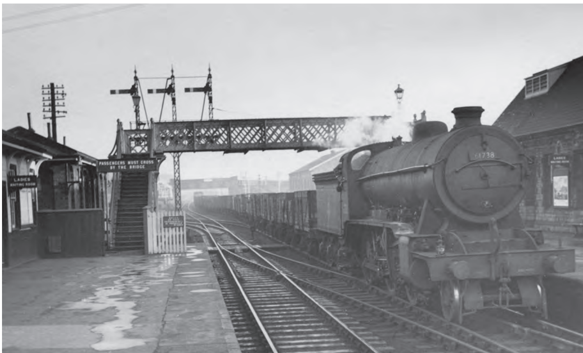
Christmas Eve 1953 at Basford North. Gresley 2-6-0 Class 'K3' 61821 threads the junction with a westbound Goods train; built in 1924 at Darlington Works and withdrawn from Immingham shed in September 1962, it was cut up at Cashmore's, Great Bridge. With the cessation of passenger services on the GNR the station closed on 7 September 1964. (M.E. Kirk/Martyn Reeve Collection)
