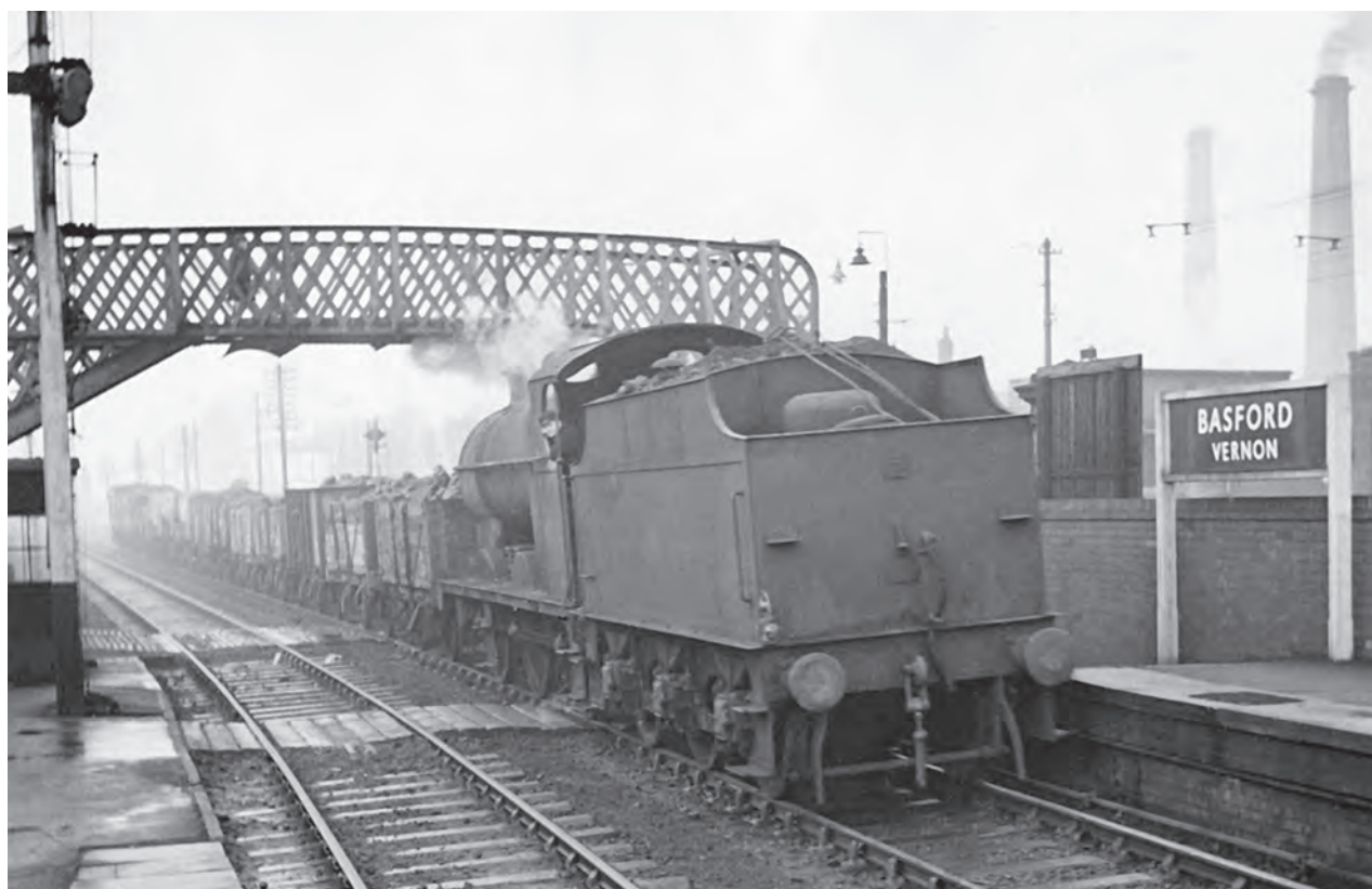
The 9.20am (SO) Basford (North)-Scarborough has just left Basford North station on 3 July 1954 behind 4-6-0 Class 'B1' 61033 Dibatag . Built in 1947 at Doncaster Works and withdrawn from Canklow shed in March 1963 it was broken up where it had begun its life, at Doncaster Works. The rear portion of the train is composed of GCR 60' saloons. (M.E. Kirk/Martyn Reeve Collection)
