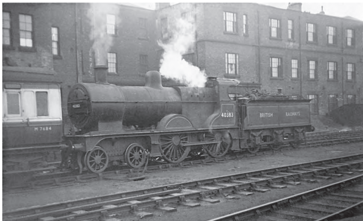
Johnson 4-4-0 Class '2P' No. 40383 is on station pilot duty at Derby on 19 January 1952. It was built in 1888 at the nearby Works and disposed of there when withdrawn from Derby shed six months after this photograph was taken. (M.E. Kirk/Martyn Reeve Collection)
