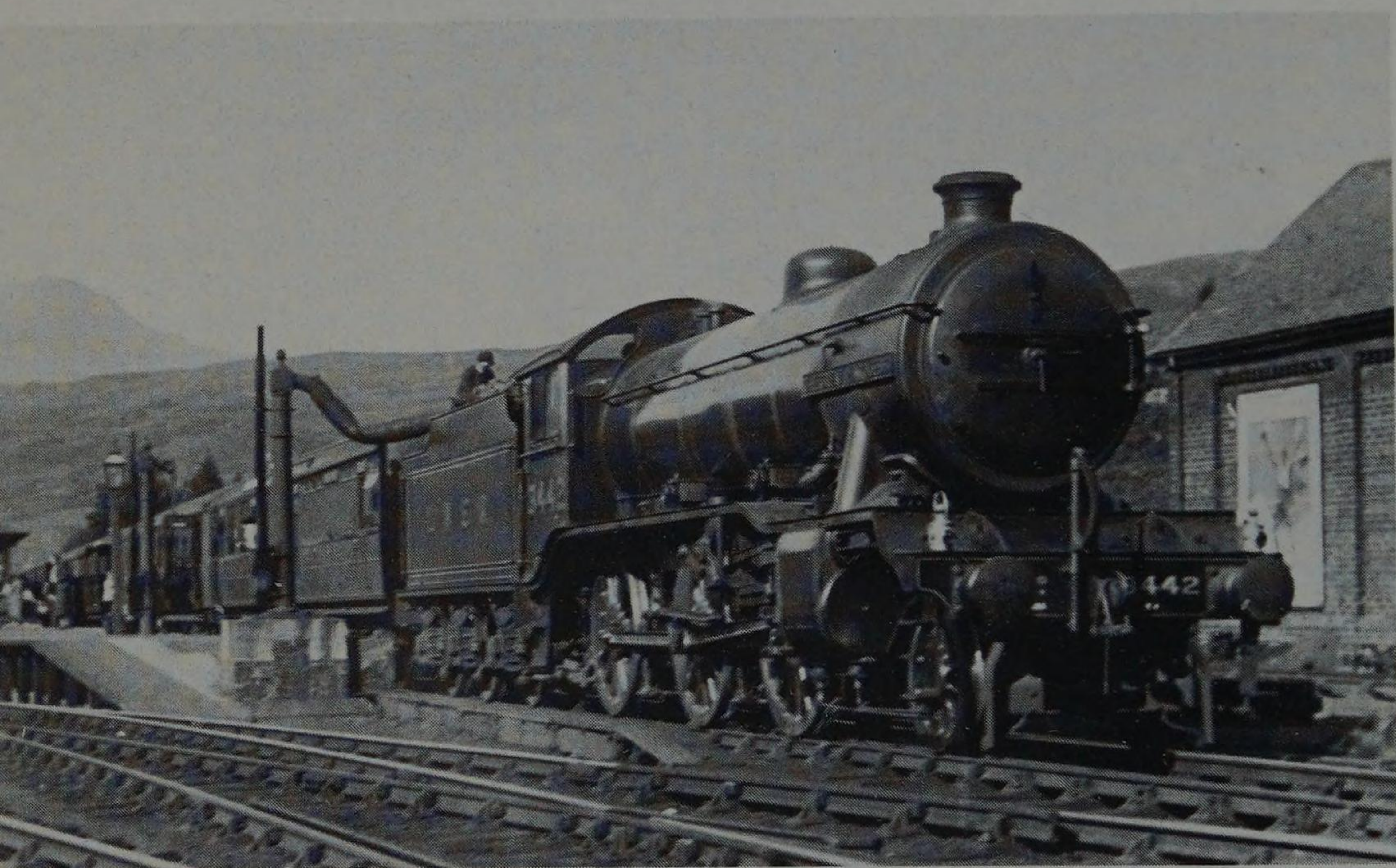
Top: The first K4 No 3441 Loch Long in original black livery at Eastfield in 1937. The steam pipe angle differs from that of later engines. Ian Allan Library
