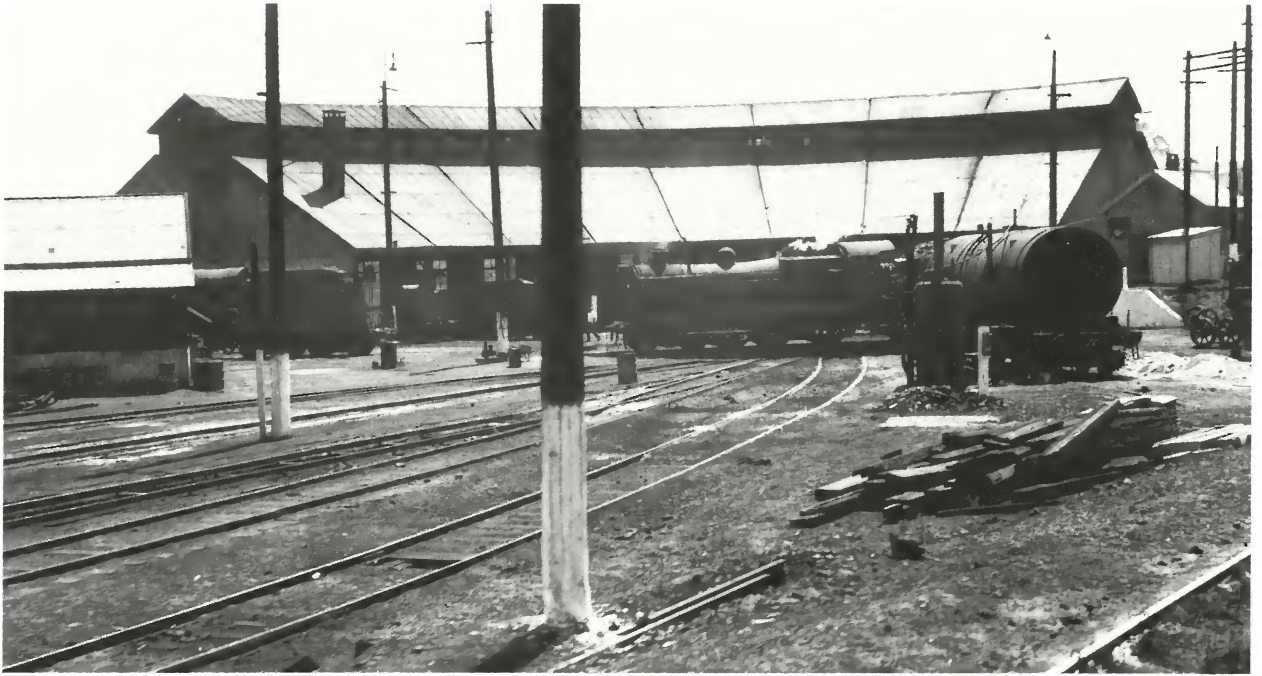
The view from a passing train, the 'North Coast Daylight Express' in October 1957. A 35 class rides the turntable, whilst to the right of the photo a mobile fuel tanker, containing bunker oil for oil-burning 55 and 59 class engines, stands on an outside shed road. A small vertical boiler is located beside the tanker, whereby steam is used to heat the thick oil to aid in rapid filling of locomotive bunkers.
