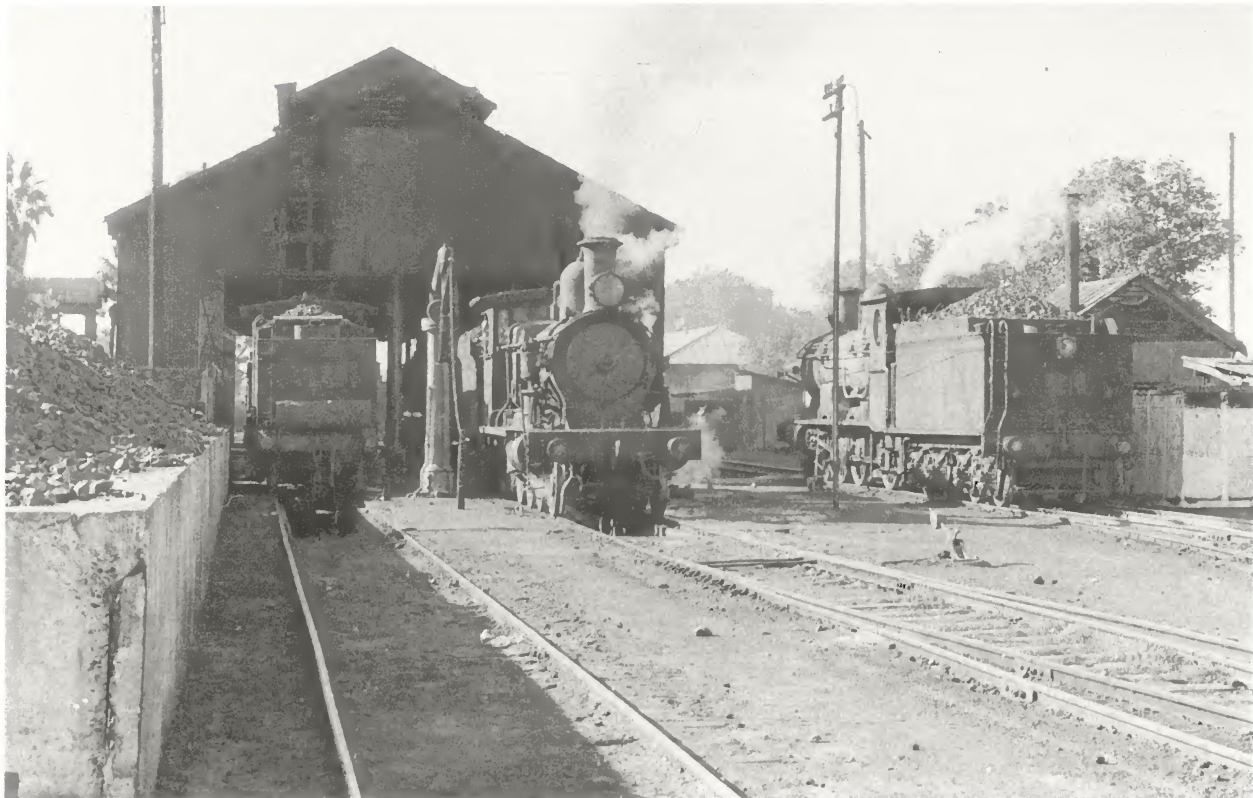
The scene at the western end of Narrandera loco showing the two road, iron shed and the coal stage at left. Standing outside, left to right, are 3028, 3082 and 3218, the P having an electric headlight fitted to the rear of its tender. 3082 is about to depart loco to take out the down passenger service to Griffith. Thursday, 18 May 1961.
