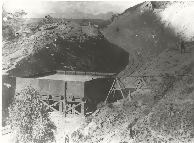
When the line was extended from Capertee to Rylstone in 1884, a water tank was erected at Brogans Creek to serve steam engines. This view, taken not long after the opening of the line, shows how advantage was taken of a low cutting to locate the tank. Although a standard water feed pipe has been fitted to the side of the tank, a more direct supply supported by trestles has been adopted instead. This view is looking south-east towards the Capertee Valley.
