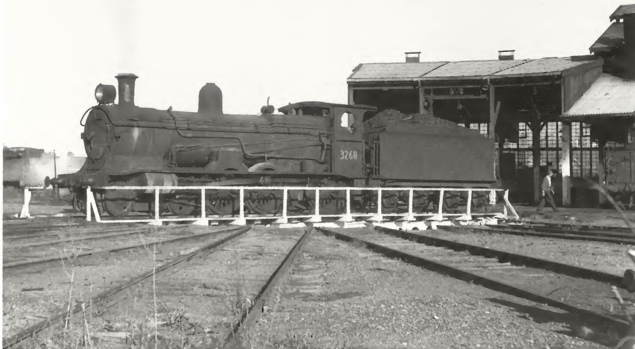
3260 on the turntable at Temora loco prior to being stabled. Earlier, 3260 had worked in No.5 Temora Mail from Cootamundra. To the left of the picture is stored 3061 and, to the right, the tender of 3285. Note 3260's original Beyer, Peacock low frame. Wednesday, 17 May 1961.
