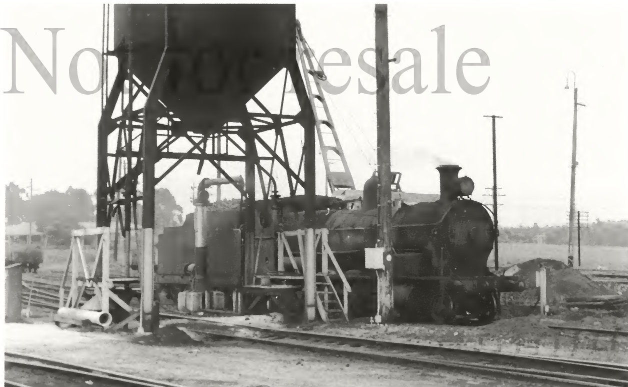
The sand tower, water column and the jib of the coaling crane surround turret-tendered 5040 in Taree loco in 1964.
