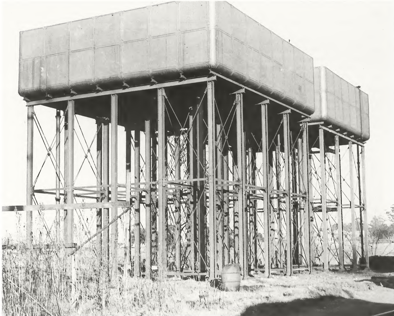
The prime source of water supply to Taree Depot, the two large elevated water tanks adjacent to the roundhouse. The tanks had been connected to the local council supply in November 1927.
