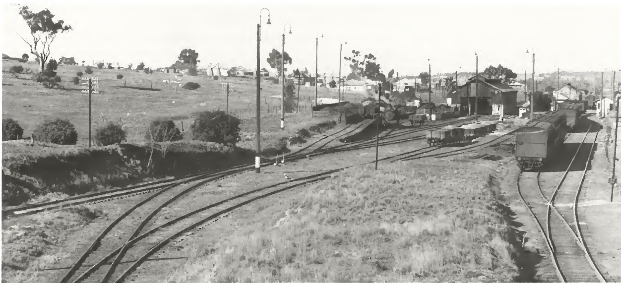
Narrandera depot viewed from the western (Hay) end, also in 1954. The road on the left of the photograph leads to the turntable, with coal stack sidings in the middle distance to the left of the shed. The carriage sidings are on the right, with the main goods yard and station out of picture to the right. SRA
