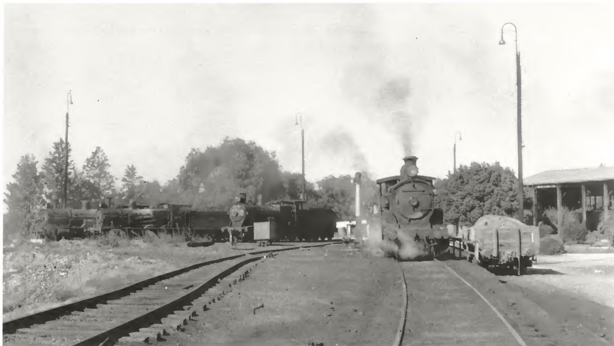
Cowra was a pleasant, compact locomotive depot. Here, from left to right, 3376, 3058, 3233 and 5487 stand out in the open on Saturday, 20 May 1961. Note the timber-constructed ash truck on right, beside the departure road. The roundhouse can be seen on right.
