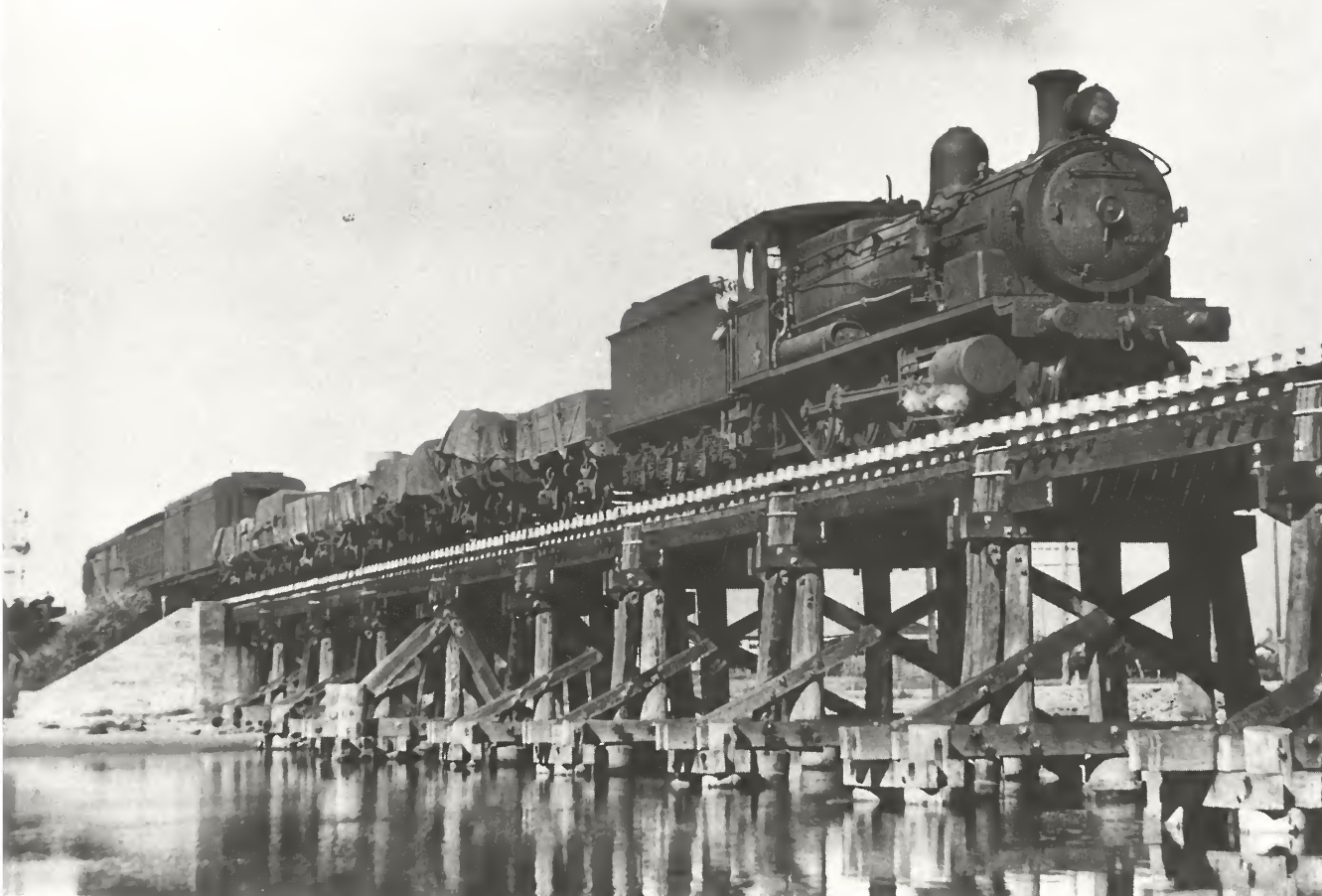
Another scene of the wooden trestle north of Coffs Harbour Station. A 53 class locomotive, complete with Laird crosshead, drumhead smokebox and small tender, heads north towards Grafton. In steam days, crews from Kempsey and South Grafton shared the goods working in this section of the Coast. SRA
