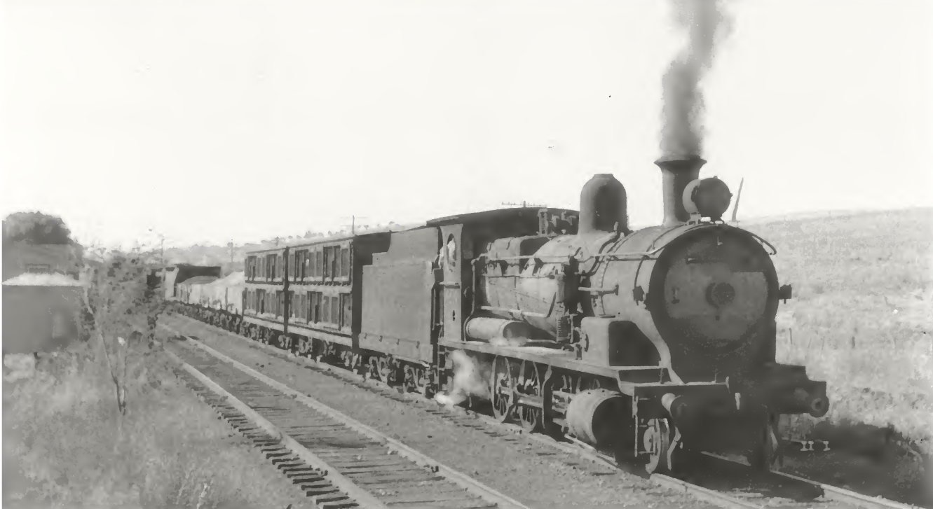
In steam days Swan Ponds was an important crossing loop between Cowra and Blayney where locomotives could take on water and de-ash. Here Bathurst engine 5445 on a Cowra-bound goods crosses No.338 Cowra to Blayney mixed, which is standing at the station at left of photo. Saturday, 20 May 1961.
