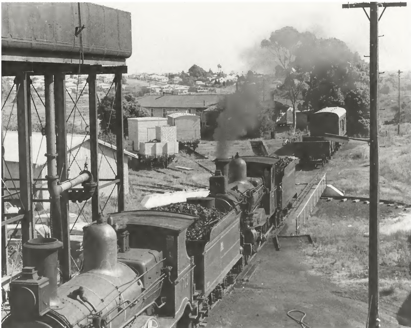
In 1967 the vintage train visited the North Coast and train locomotives 1243 and 1709 were serviced in the former Kempsey depot area. The roundhouse has been demolished but pits, roads and turntable were still usable. Part of the barracks can be seen beyond the work vans.
