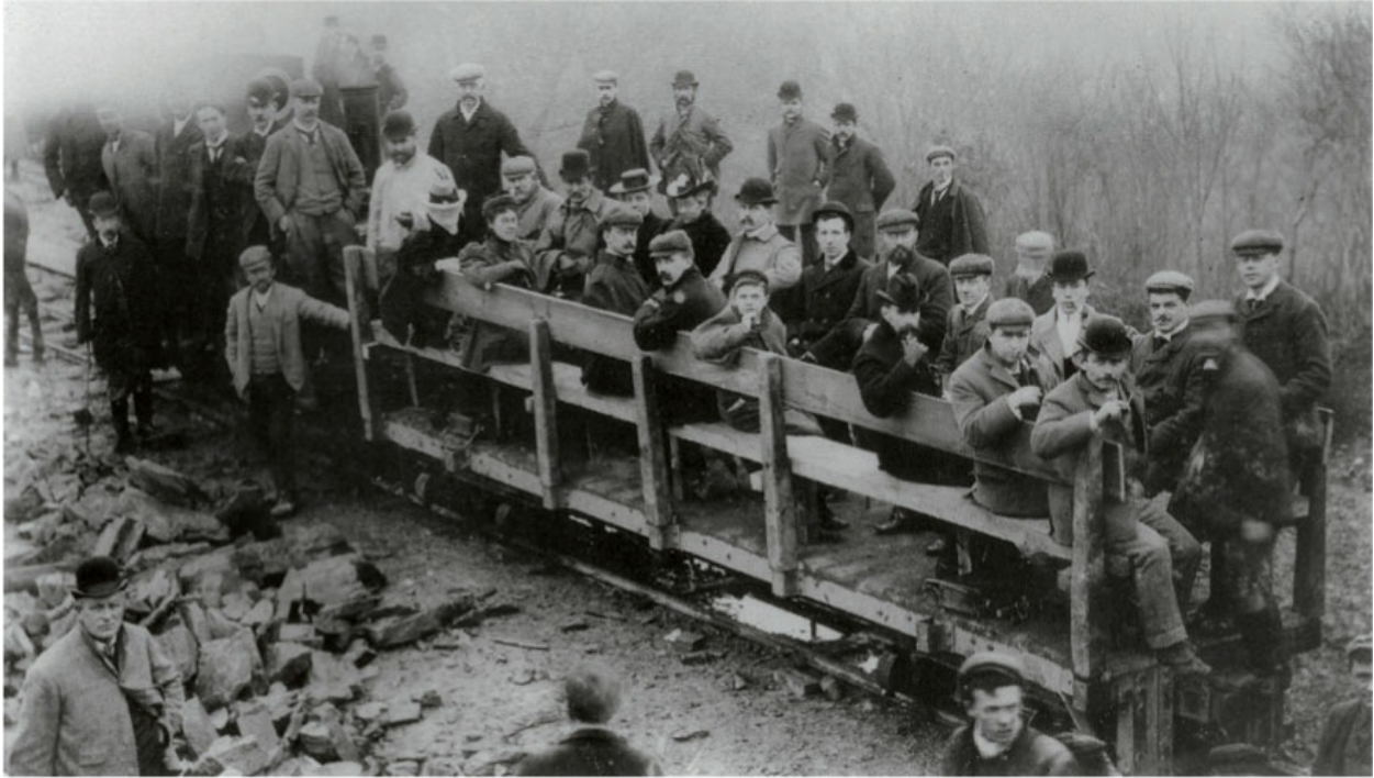
The bogie bolster wagon, seen here with longitudinal benches fitted. This wagon transported visitors to view progress with the construction works. MAJOR, DARKER & LORRAINE
