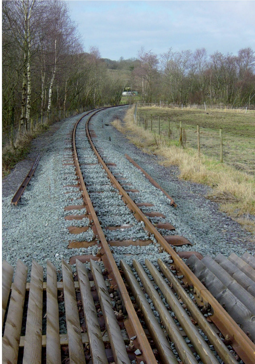
The rebuilt Welsh Highland Railway uses new rail of 30kg/m, about 60lb/yard.
