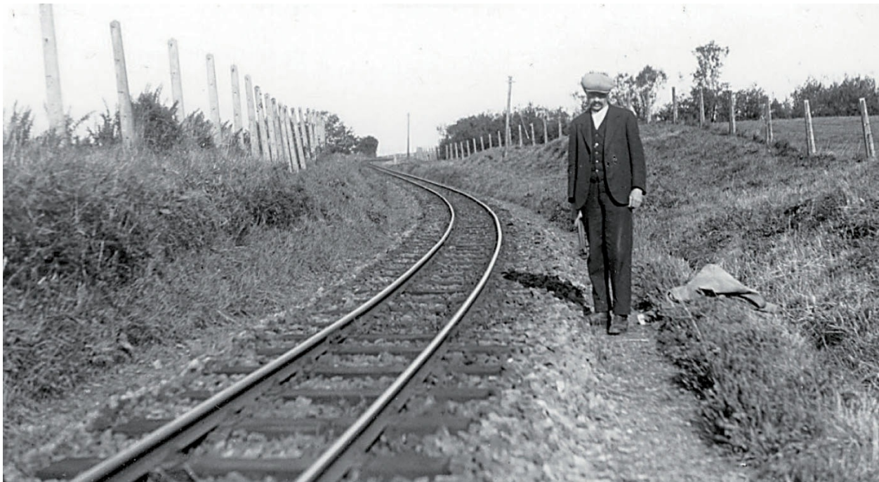
The 1ft 11½in gauge track with 40lb/yard rail, near Parracombe, Devon. W. W. DUNNING
