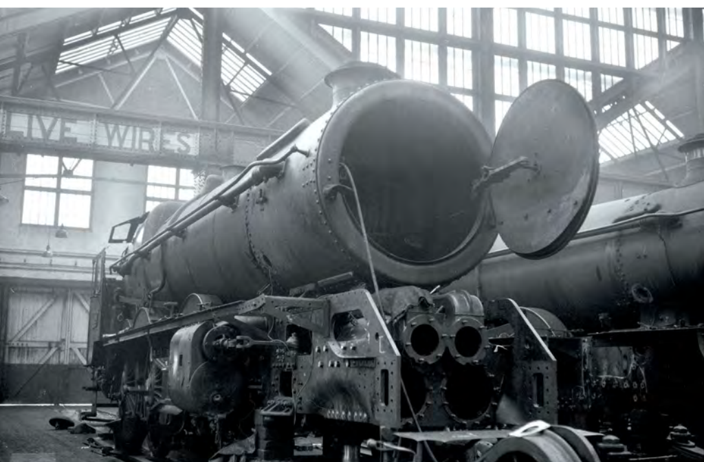
No 6022 King Edward III is seen inside Swindon Works 'A' shop in the middle of a Heavy General repair on 5 October 1955. With the inside cylinder exposed, the layout of the cylinders is apparent, and the rocking levers from the inside valves to the outside one can also be seen. At this time the 'Kings' were going 18 to 20 months between major attention, but light repair and casual repairs occurred more often. By this date No 6022 was credited with having run over 1.3million miles almost exclusively on Top Link duties, a feat other '8P' class locomotives rarely achieved.
