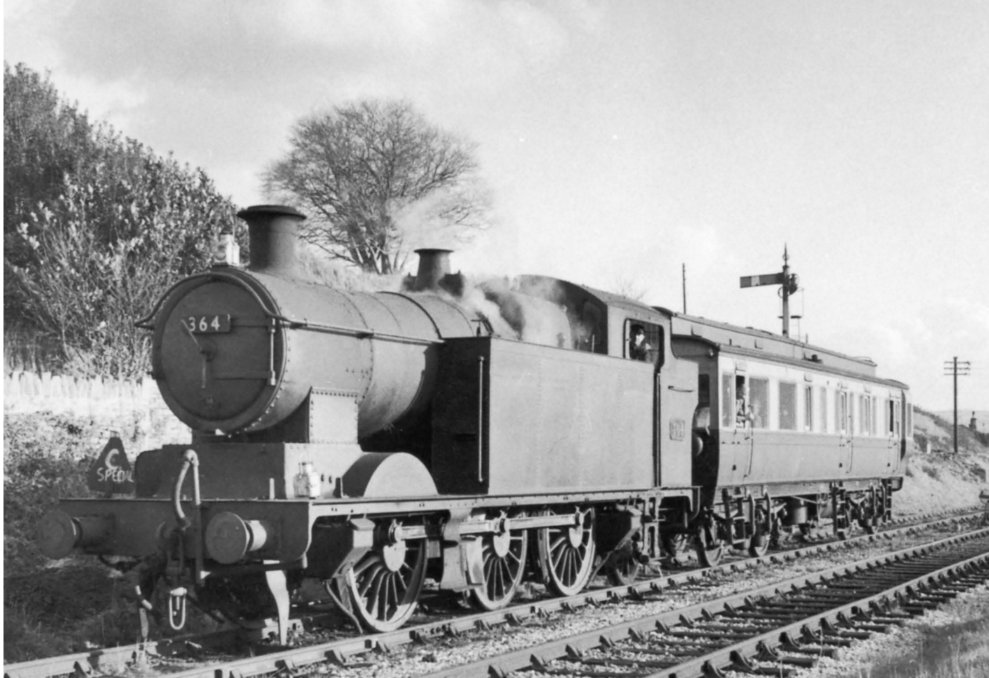
Former Taff Vale Railway 'A' class 0-6-2T No 364, one of 65 engines of the class that survived into BR days, is seen here working an Officers' special train near Hirwaun on the Vale of Neath line in December 1954. The GWR rebuilt these engines with Standard No 10 boilers which resulted in excellent steaming capabilities, and No 364, pictured here, shows evidence of the conversion at Swindon Works by the squared-off top to the side tank as opposed to the rounded top of Caerphilly Works.
