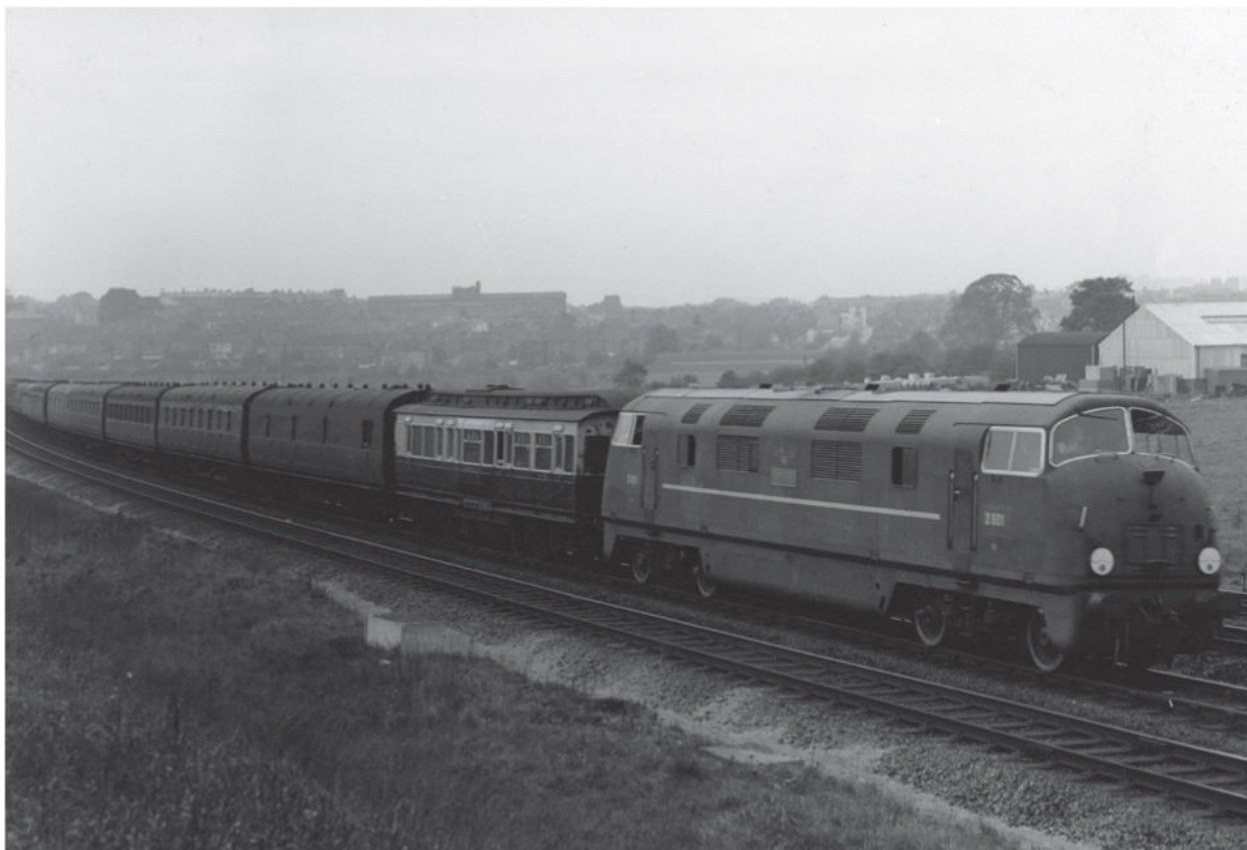
Swindon-built D801 Vanguard on test near Bristol. Like the D600s, most D800s were named after British warships. The bogie problem mentioned in the text had been solved by 1963.
