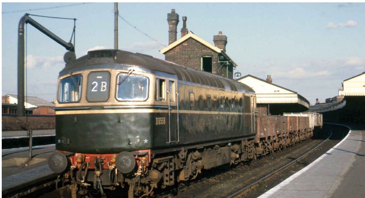
‘Type 3’ referred to the 1,500– 1,999hp power range. Between 1960 and 1962, BRCW built ninety-eight such locomotives for the Southern Region – including D6556, seen at Salisbury in 1964.
