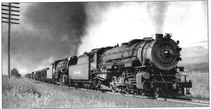
RIGHT: Two well-matched 'Mountain'-type engines of the Denver & Rio Grande Western carry a northbound freight of 66 cars near Pikeview, Colorado, in August 1941. The Rio Grande was one of several western lines that painted engine fronts and fireboxes silver.
