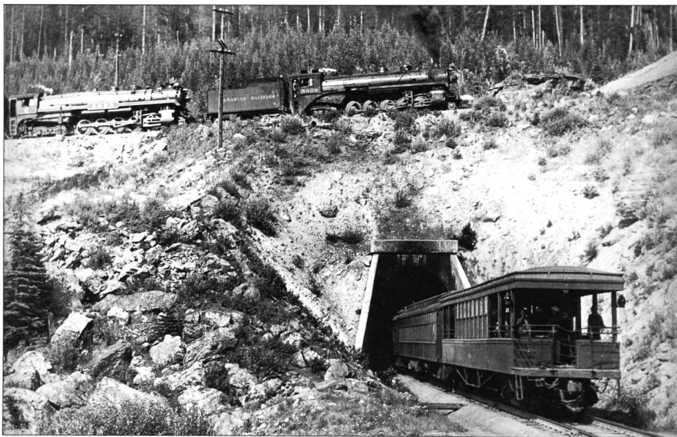
BELOW: The Canadian Pacific's train, the Trans-Canada Limited, ran between Montreal and Vancouver via the spectacular Canadian Rockies. En route are the twin Spiral Tunnels, each carved in a loop within opposite mountains. With a 'helper' engine in front and a special open-air car on the rear, this is one train, artfully posed.
