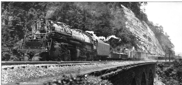
LEFT: On the Baltimore & Ohio, a freight comes downgrade over Tray Run Viaduct in 1949. There is some brakeshoe smoke back in the train; a trail of steam comes from the engine's electric dynamo. No. 7609 is a huge, four-cylinder EM-1, among the most powerful steam locomotives anywhere.
