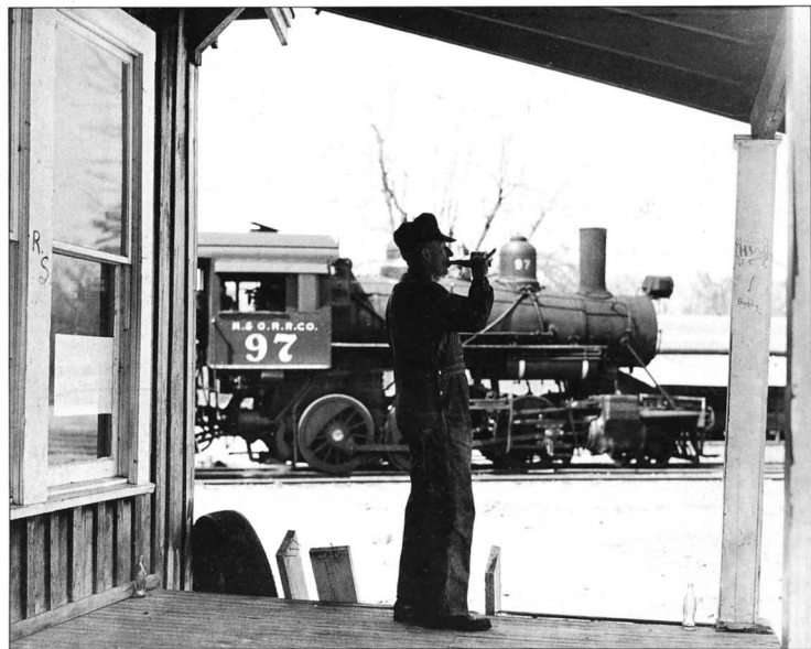
RIGHT: Before the era of mobile radios, crew members on moving trains got their train orders 'on the fly' as this freight conductor on the Western Maryland Ry. is doing in this Frank Quin photo made at Deal, Pennsylvania in 1940. The train's engineer has already picked up his copy from the order hoop. Another engine waits in the siding; a young lad watches from his bike.
