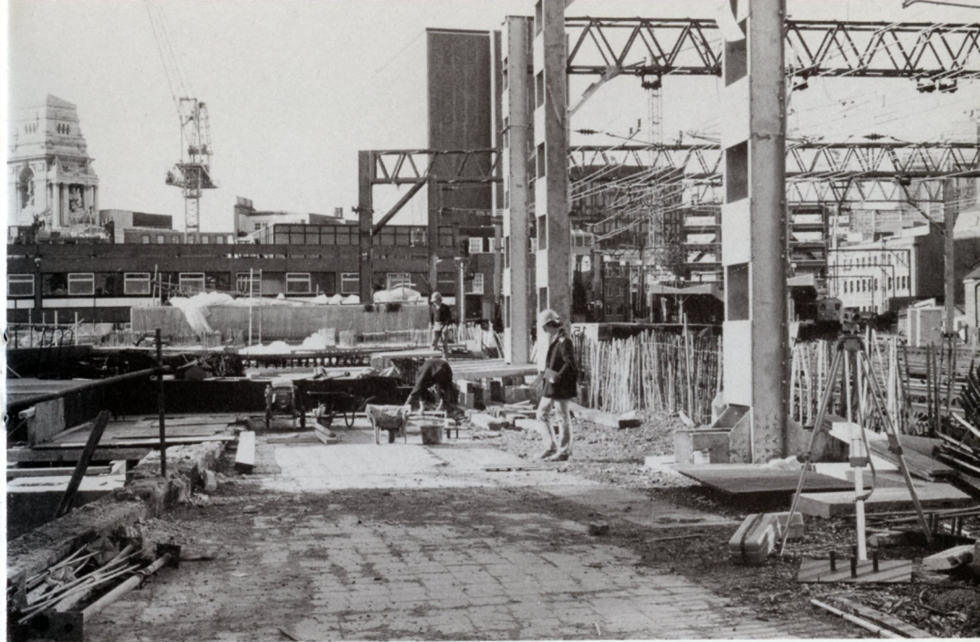
An impression of the difficulty of shoe-horning a new railway into an old urban fabric is given by this westward-looking view of the Tower Gateway terminus site in November 1985. The British Rail electrified lines on the right impose their own limitation on overhead clearances, whilst the existence and then the partial demolition of the multi-storey car park to the left of the picture posed further restrictions.
