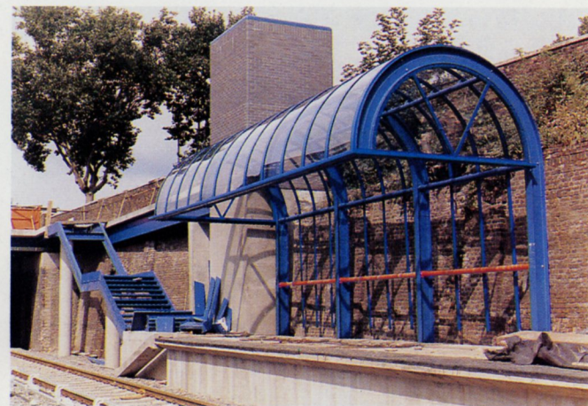
All Saints station with glazed canopies in place and the stairs to East India Dock Road being assembled in August 1986.
