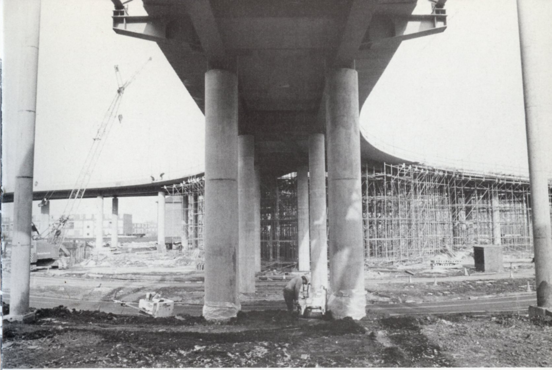
North Quay triangular junction, the heart of the initial railway, in February 1986. The great height of the junction above local road level is necessary in order to give clearance for pleasure craft in the West India Docks, which are immediately behind this camera position. The city route curves off to the left (west) and the Stratford route to the right (east).
