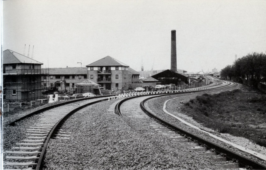
Re-using former railway land, new DLR tracks have already been ballasted beside East Ferry Road (right) on the old Millwall Extension Railway route south of Glengall Grove (background right) and Crossharbour station. New houses built on the western side belong to the Clippers Quay development beside part of the former Millwall Docks.
