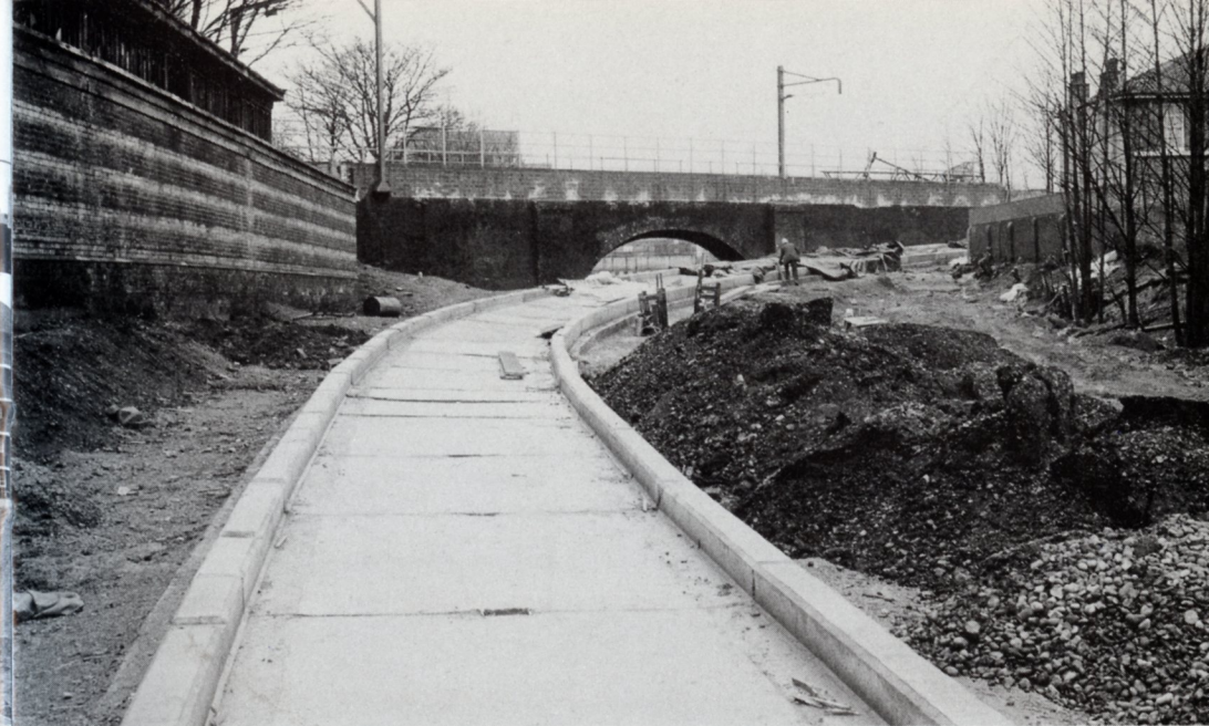
Bow Curve is a classic example of the ability of Light Rail to weave around existing structures where orthodox rail systems would need excessive demolition and land take. Here the DLR is changing direction from a north-south axis to an east-west one without destroying nearby residential property and in a situation where other British Rail lines must continue operating. In March 1986, the new line climbs and curves towards Stratford, right of picture.
