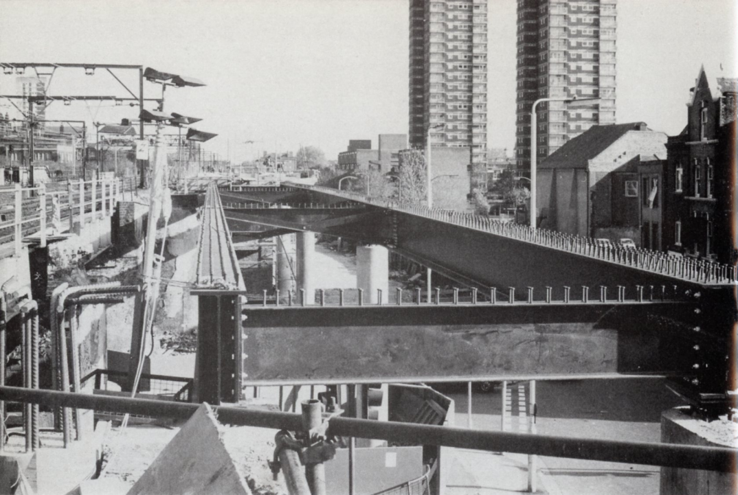
Steelwork for the future bridge decking in place over the crossroads junction of Cable Street (receding into the distance and to the east), Dock Street to the south (right of picture), Royal Mint Street (near camera position) and Leman Street (left of picture). Prominent on top of the steelwork in this December 1985 view are the bolt head reinforcements around which the wet-pour concrete decking will be added.
