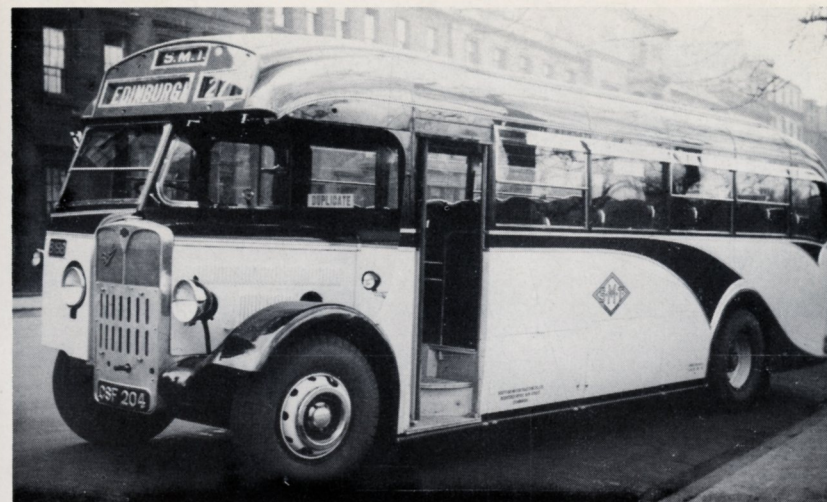
49. The A.E.C. "Regals" of 1939 had front entrance 35-seat bodies by W. Alexander painted in the cream livery. Those 1940 seated 39 and were also in the cream livery, but on them the trim was blue; B198 shown here is one of the 1939 lot.
