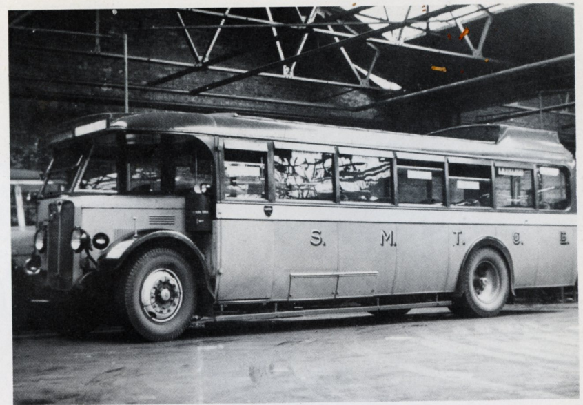
29. The 1931 coaches were A.E.C. "Regals" with 28-seat Cowieson bodies. B10 is shown.
