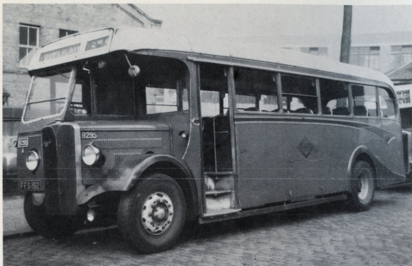
55. The first post-war additions to the fleet in 1946 and 1947 were A.E.C. "Regals" with 35-seat bodies in cream livery. The 1946 bodies were by Duple, the 1947 ones by W. Alexander. B295, one of the latter, is shown.
