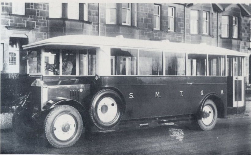
17. Two Albions were 32-seat saloons with half-cabs. These were later numbered A43-4.
