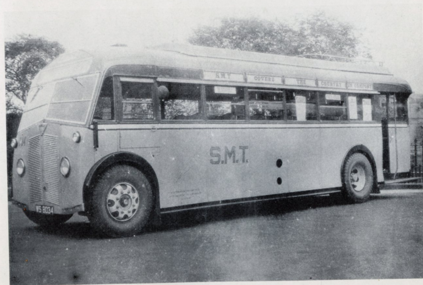
42. There were also sixty Leyland "Cheetahs" with 36-seat full-front rear entrance bus bodies by W. Alexander in 1936. This one is T34.
