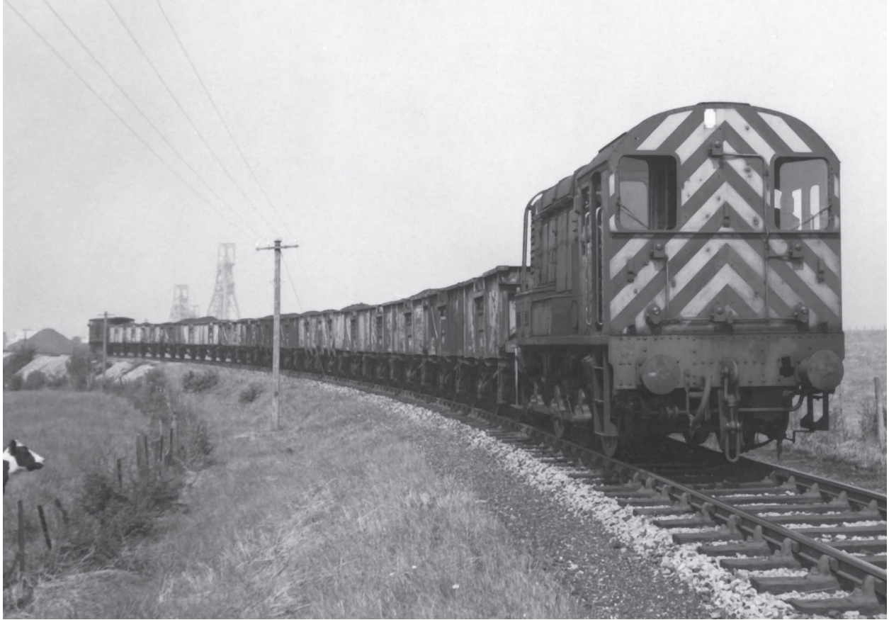
Five years later, on 17 July 1964, 350 HP 0-6-0 diesel mechanical shunter No. D4102 runs in reverse, hauling a similar train of loaded 16-ton coal open wagons from Tilmanstone Colliery, seen in the background and Shepherdswell exchange sidings. (R.F. Roberts/Stephenson Locomotive Society)
