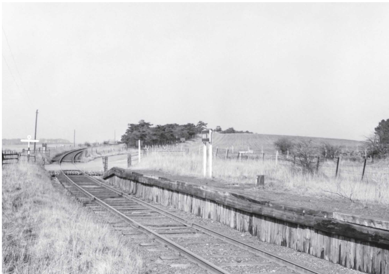
Knowlton Halt looking towards Shepherdswell on 3 March 1951, with its crude timber platform edge and facing and its lack of a basic shelter or seat for any potential passenger. This was the scene two and a half years after the last passenger train, the station name board is still intact and the platform is still free from grass or any dereliction. (Dennis Cullum, Lens of Sutton Association)
