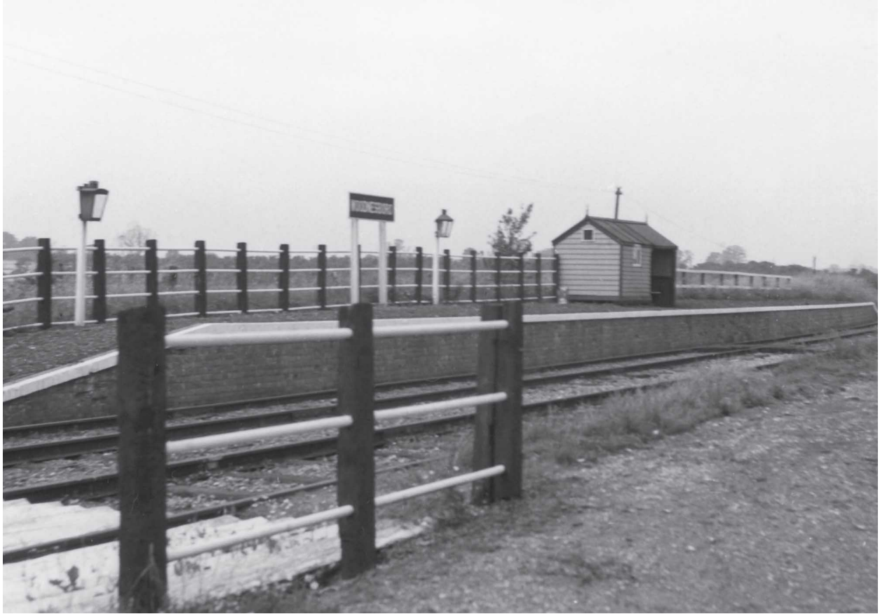
Woodnesborough station, c1936, showing the platform, timber building and steel four rail fence at one end and the two rail timber fence at the other. The station has recently been painted and tidied up in this pre-war picture, probably to try and win back some passengers from the local buses. ( Author's Collection )
