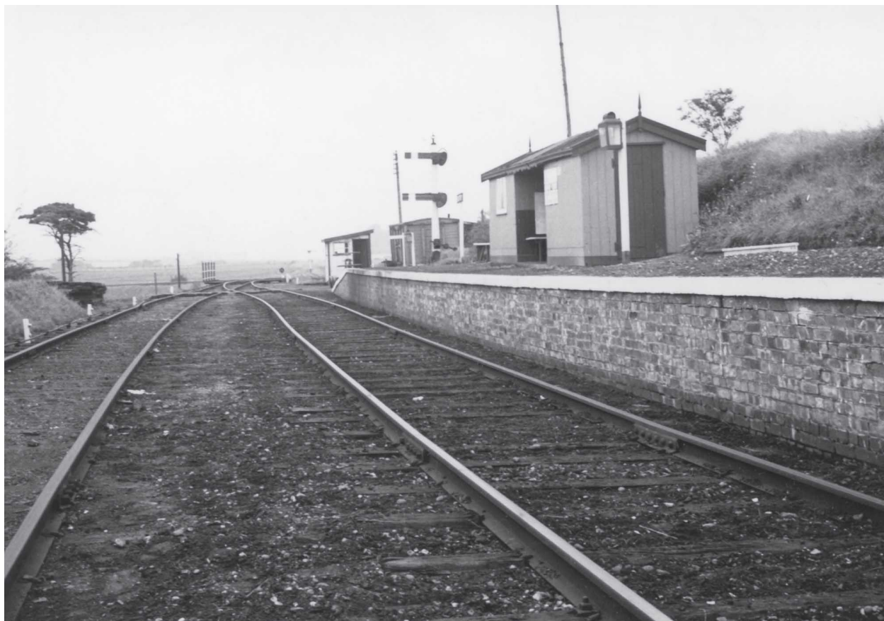
Eastry station looking towards the junction on 24 September 1938, this picture clearly shows the buildings and the two armed signal controlling the lines to Wingham and the Richborough branch. ( R.F. Roberts/ Stephenson Locomotive Society )
