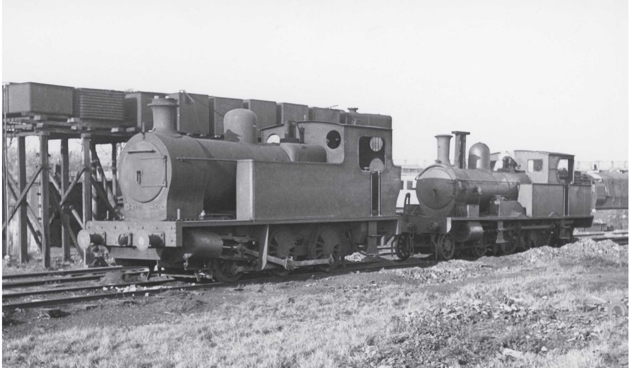
Locomotives No. 4 and No. 5 stand on a storage road near the water tanks, at the shed, c1930; the watering facilities seem to be a rather basic arrangement, with iron tanks supported by bulks of timber, in a long row. ( Ivor Gotheridge Collection )
