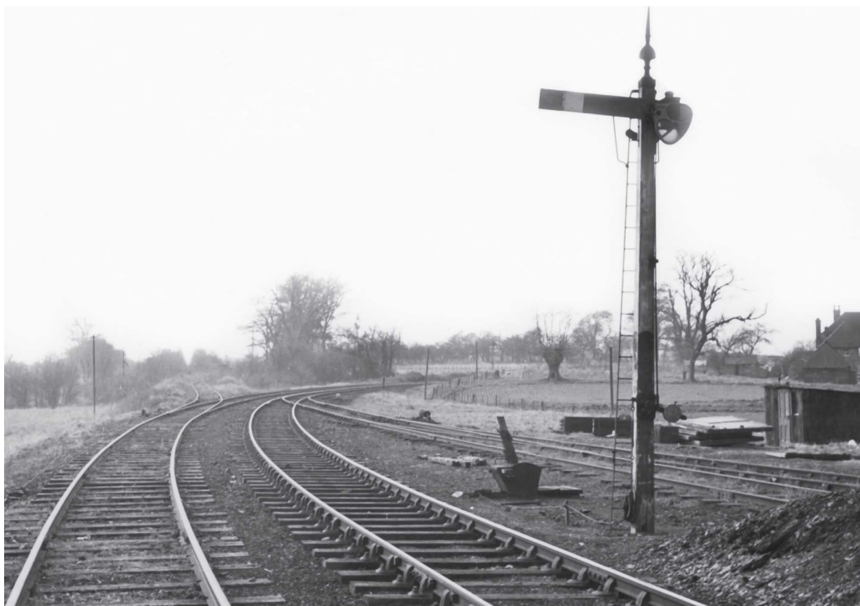
The junction at Eythorne, looking back towards Guilford Colliery, on 3 March 1951; this picture shows the track arrangement, for the station goods yard and the loop, with the derelict Guilford Colliery branch running off to the far left. ( Dennis Cullum, Lens of Sutton Association )
