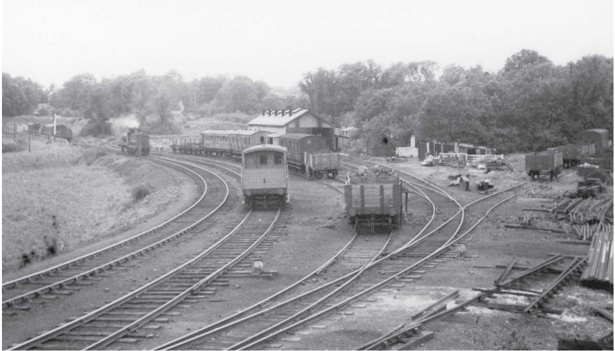
A clear view of the trackwork at the shed, showing the points and sidings fanning out from the Eythorne end of the yard, c1938. There seems to be less clutter in this picture, with fewer derelict carriages and wagons on view. In the distance, an 01 class simmers at the approach to Shepherdswell station and stock waits in the station to form the next train to Canterbury Road. ( Ivor Gotheridge Collection )
