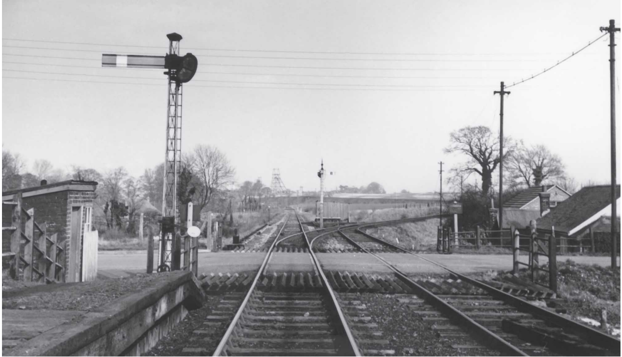
The junction for the branch to Tilmanstone Colliery pictured here on 13 March 1951, showing the signalling arrangements with lower quadrant signals and the track layout, heading off to the right towards the colliery and the main line to Canterbury Road going off into the far distance. ( Dennis Cullum, Lens of Sutton Association )
