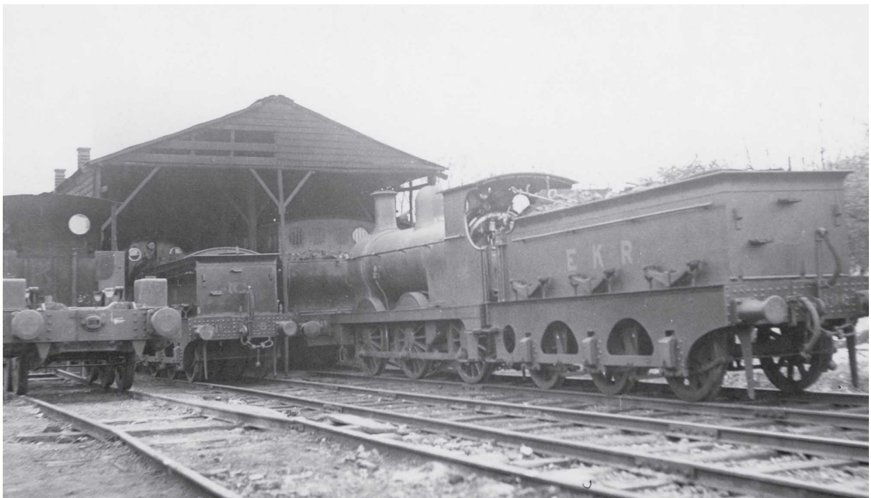
EKR No. 2 Walton Park at Shepherdswell locomotive shed and works on 18 July 1936, while undergoing a heavy overhaul. The shed building is in a rundown condition, with most of the far wall missing, while locomotives 4 and 6 can be seen in the picture. ( Photomatic )
