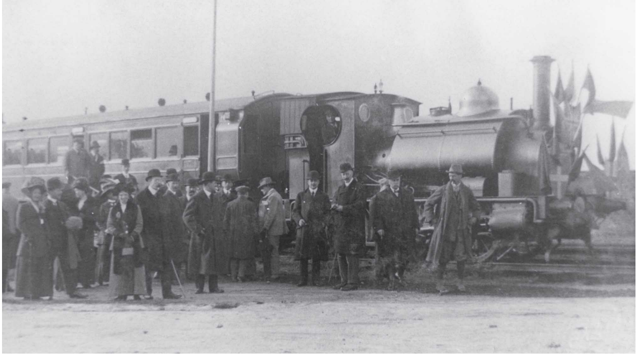
A shareholders' special train headed by Fox Walker constructed saddle tank No. 1, on 27 November 1912. The carriage behind the locomotive is a former Kent & East Sussex bogie brake vehicle, which was transferred to the East Kent Railway, to provide the line's first passenger vehicle. This carriage was originally Kent & East Sussex Railway No. 17, being constructed by R.Y. Pickering in May 1905 and numbered 1, on the East Kent Railway, withdrawn by British Railways in 1948. ( Ivor Gotheridge Collection )
