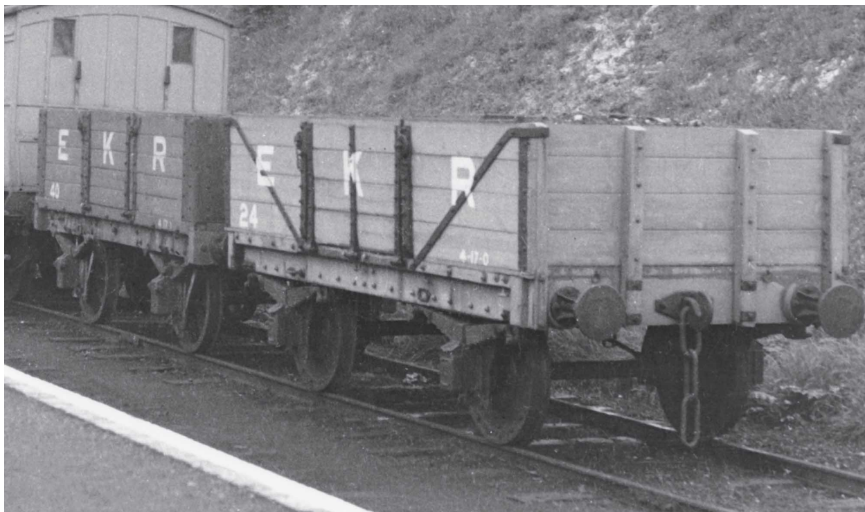
A pair of former SER four-plank open wagons Nos. 24 and 40, here seen on the siding at the East Kent Railway station at Shepherdswell, August 1937. Both are painted in East Kent Railway light grey, with black ironwork, No. 24 having Mansell wheels. ( J.W. Sparrow )
