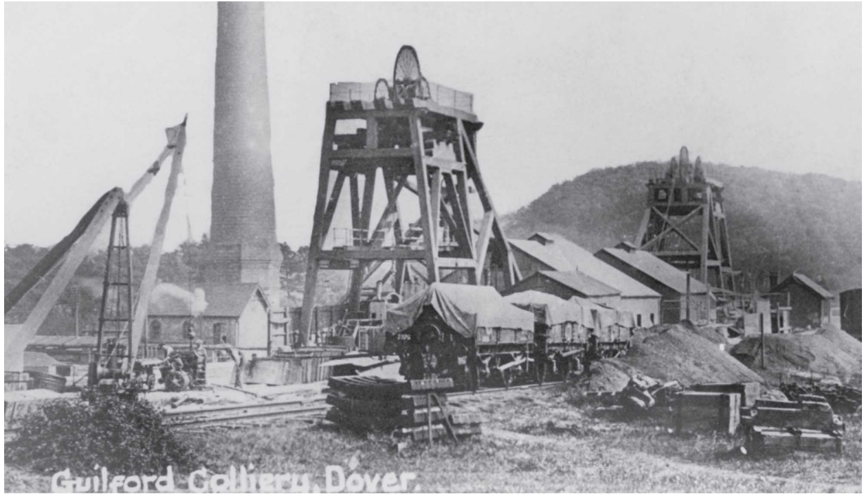
Guilford Colliery, c1912, showing the rail connection and wagons of materials waiting to be unloaded for the construction of the colliery buildings and mining machinery. By this time, the pit head gear is in place and the chimney for the boiler house is already erected, ready for the main buildings to be constructed. ( Author's Collection )
