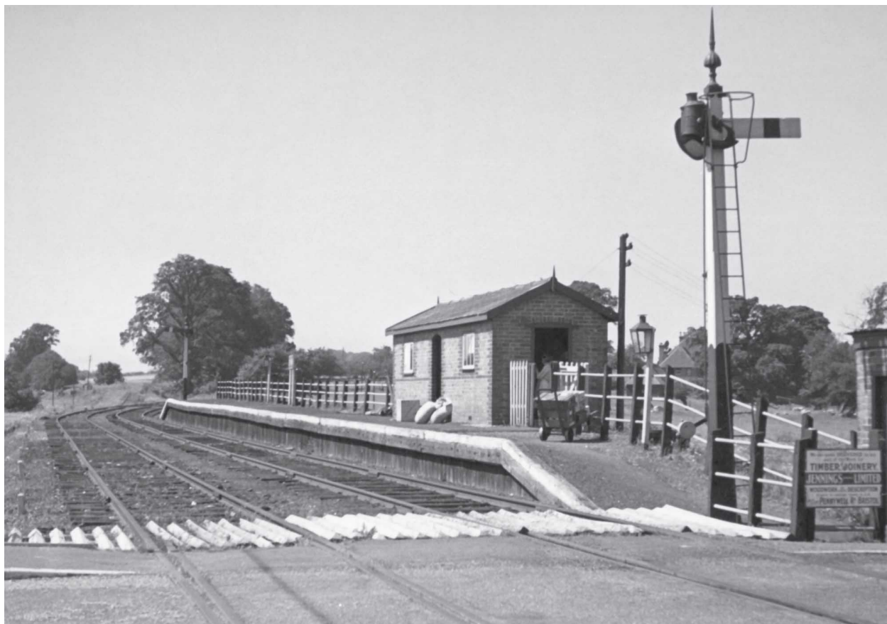
Eythorne Station looking towards Shepherdswell on 29 July 1939. This picture shows the station layout to good effect, with the loop and the substantial brick building and long platform, note the wooden posted lower quadrant signals and the oil lamps on the platform. (S.W. Baker)
