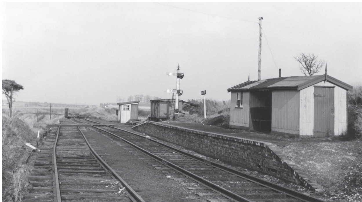
Eastry station from the other direction, looking towards the junction. This picture shows the double armed signal controlling the lines to Richborough Port, far right and the line to Canterbury road far left. The grounded van body and signal ground frame shed are of interest; by this time, British Railways had taken over and removed the point nearest the road overbridge, thus making the former loop a siding, 13 March 1951. ( Lens of Sutton Collection )
