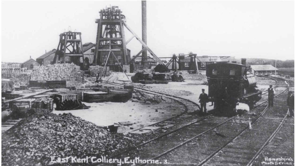
An early photograph taken during the construction of Tilmanstone colliery, c1912, with locomotive No. 1 standing in the colliery yard. In this picture, the locomotive has a makeshift rear spectacle plate to the cab made of timber and the pit head gear is well on the way to completion. ( Local Postcard )
