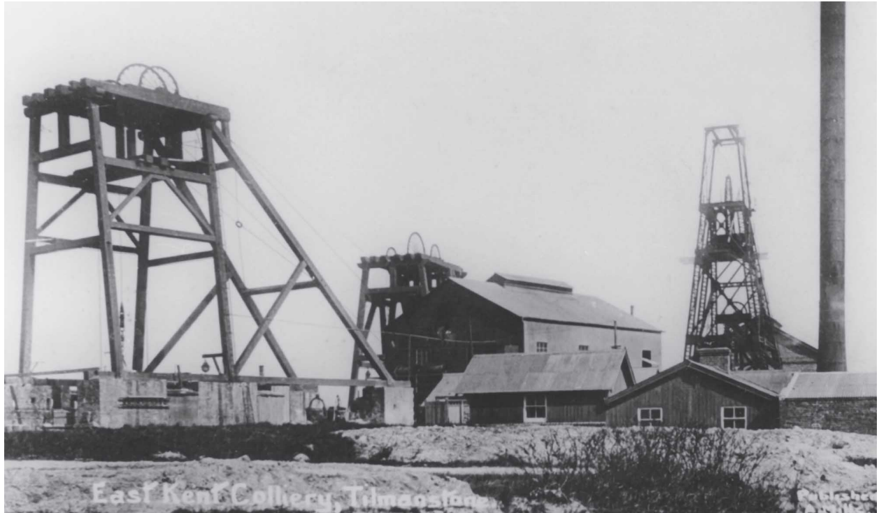
The pithead gear at Tilmanstone Colliery, c1930, showing the original timber framed winding tower and the later more modern steel constructed winding equipment. ( Local Postcard )
