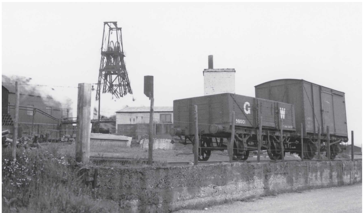
The pithead gear at Tilmanstone Colliery, c1930, showing the original timber framed winding tower and the later more modern steel constructed winding equipment. ( Local Postcard )
