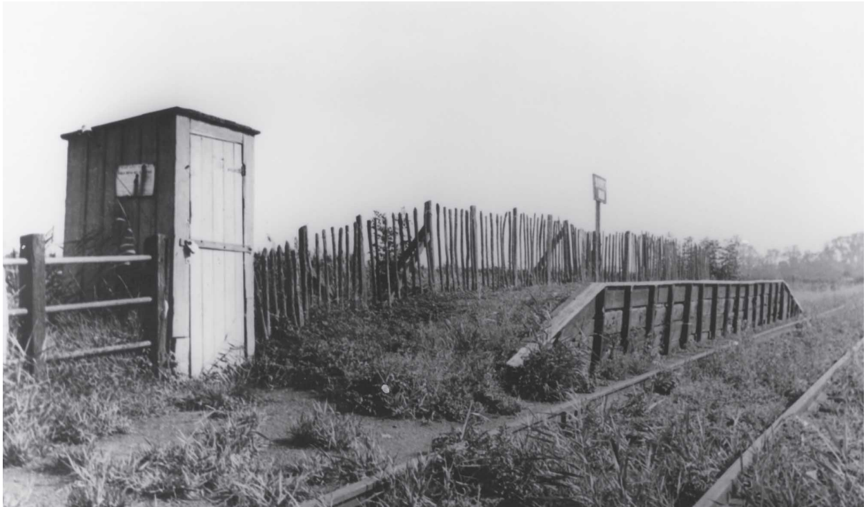
A forlorn looking platform and ticket hut at Sandwich Road Halt, with grass growing between the sleepers and a feel of dereliction, c1936. The block section from Poison Cross Halt to here, had a token, with a brass plate on it, which read Poison-Sandwich. ( R.K. Blencowe Collection )
