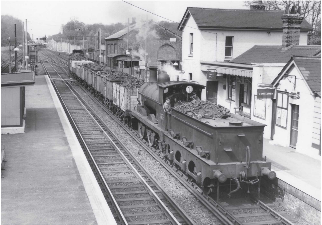
01 class No. 31258, passes through Shepherdswell main line station, with a train of mineral wagons for Dover, in April 1960. By this time, the third rail was already laid and waiting for the next phase of the Kent coast electrification, which would be the death knell for South Eastern steam traction in 1961. ( Derek Cross )
