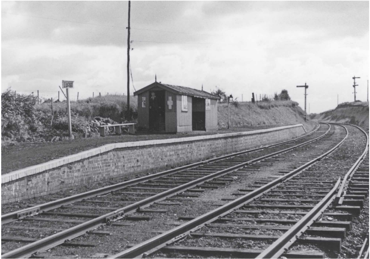
A general view of Eastry station, on 15 September 1936 showing the platform, timber building and run around loop, with its heavy poundage track, note the catch point on the middle right. This picture also shows the signalling arrangements for the line to Shepherdsweil in the far distance. ( J.H.L. Adams )
