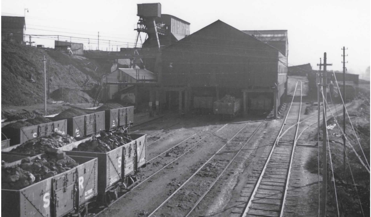
Southern Railway eight-plank open wagons, loaded in the colliery yard at Tilmanstone, c1936. The large large building in the background is the washery. ( Ivor Gotheridge Collection )
