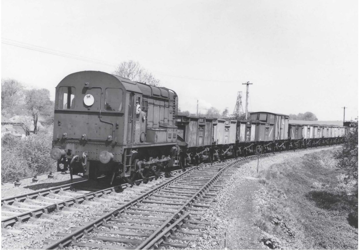
350 H P 0-6-0 Diesel Mechanical shunter No. D3044 heads a train of 16-ton mineral wagons and a solitary van, at the junction of the Tilmanstone colliery branch at Eythorne in April 1960. Both classes 08 and 09 were used on the branch in British Railways days, for shunting and trip working of these colliery trains. ( Derek Cross )
