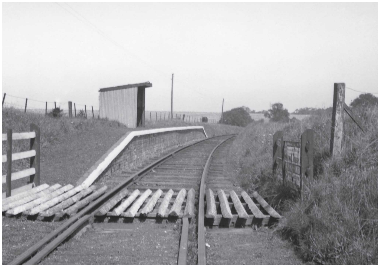
Elvington station on 2 September 1938, showing the brick platform with its basic waiting shelter, looking towards Eastry. The station is in good condition and well kept; note the cattle grid in the foreground, a feature of most of the stations and halts on this line. ( R.S. Carpenter Collection )
