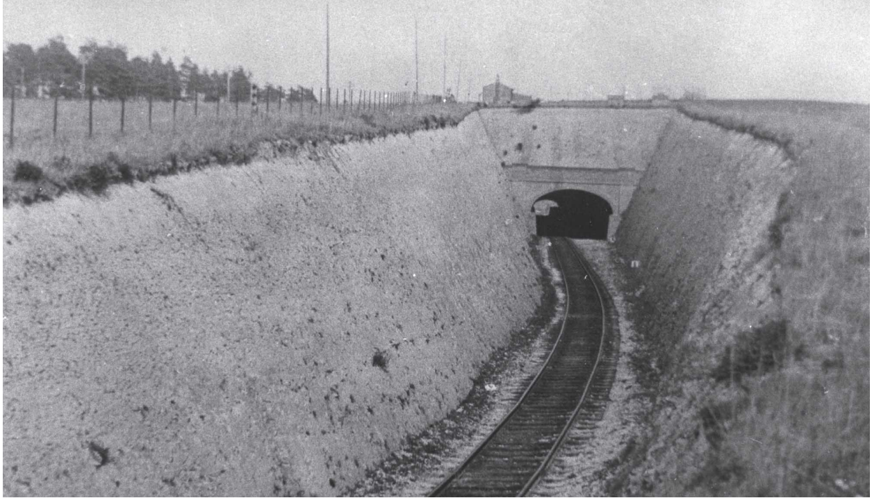
The approach to Golgotha tunnel, from the Eastern end, c1913, showing the freshly cut chalk cutting and the portal for a double track line, which was never constructed. The alignment on the right of the picture had large blocks of uncut chalk right through the formation of the tunnel, being bricked along the ceiling and rough cut in chalk along the sides. ( Ivor Gotheridge Collection )
