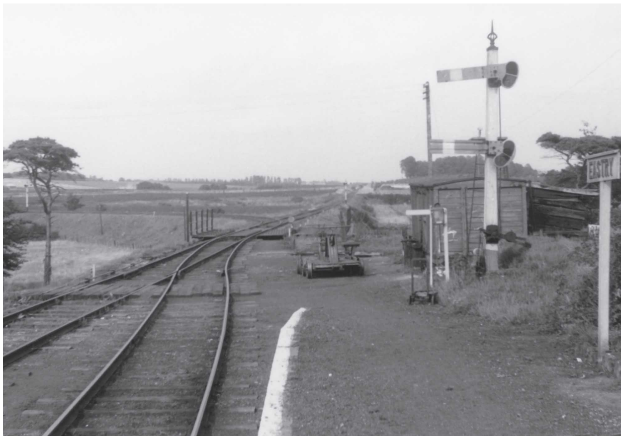
A further view of Eastry taken from the platform, c1936, looking towards the junction, clearly showing the double arm signal and a pump trolley by the grounded van body. ( Author's Collection )
