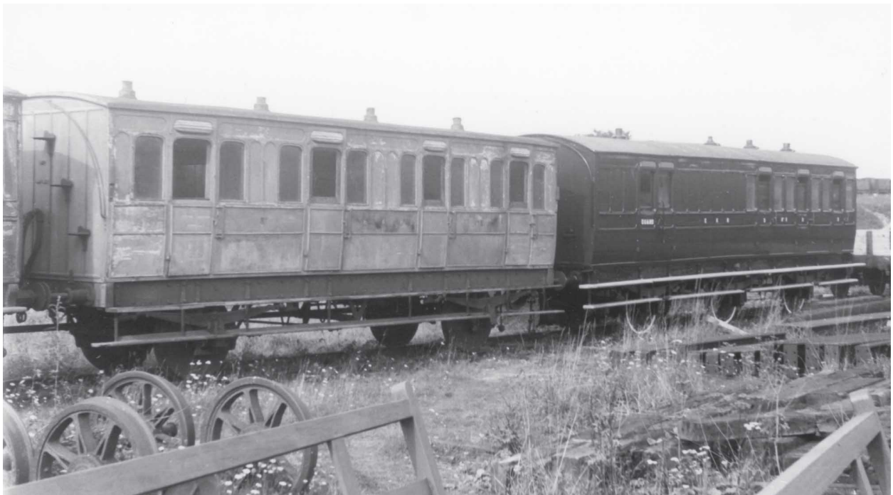
Carriage No. 4 was an ex-Midland Railway six-wheel first, third compartment vehicle constructed at Derby in 1882. Originally a slip carriage on the Midland Railway, it was purchased for £180 by Colonel Stephens 1919 for use on the East Kent Railway, surviving until 1948, when it was scrapped. ( Photomatic )
