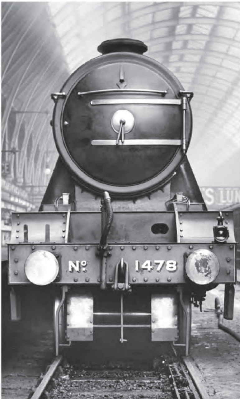
When first built, the original 'A1s' had quite a different look to later on – as they were constructed to the generous Great Northern loading gauge and so could have, for example, larger chimneys. This is No 1478 Hermit (later No. 4478) after arrival at King's Cross with an express from Leeds in 1924. F R HEBRON/RAIL ARCHIVE STEPHENSON
