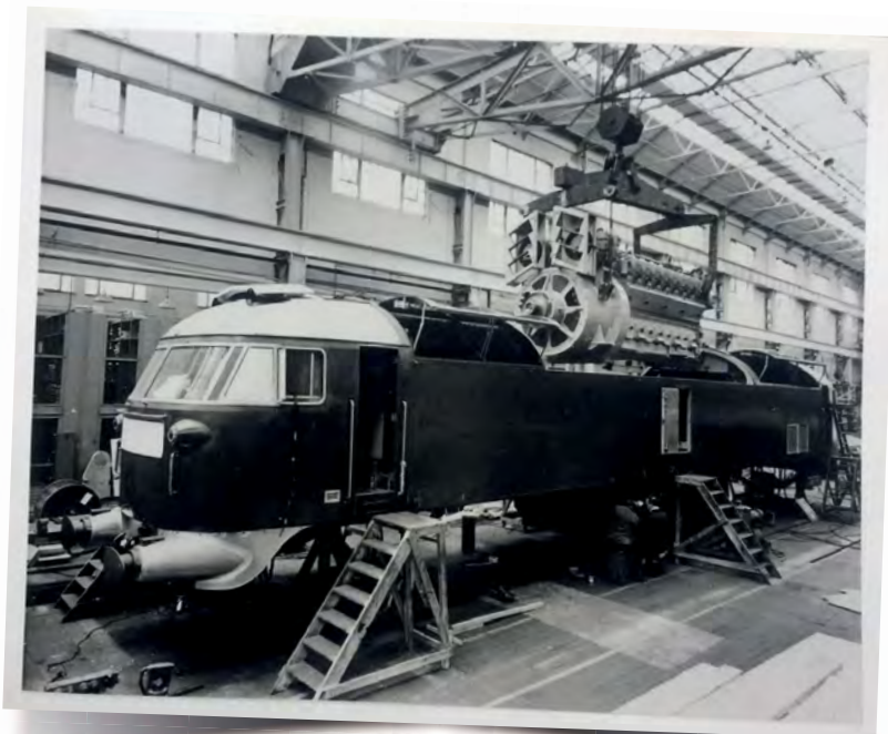
LEFT: Kestrel under assembly at Brush's Falcon Works in 1967, with the 4,000hp Sulzer powerplant being lowered into the engine room. (Brush via Ian MacLean)
