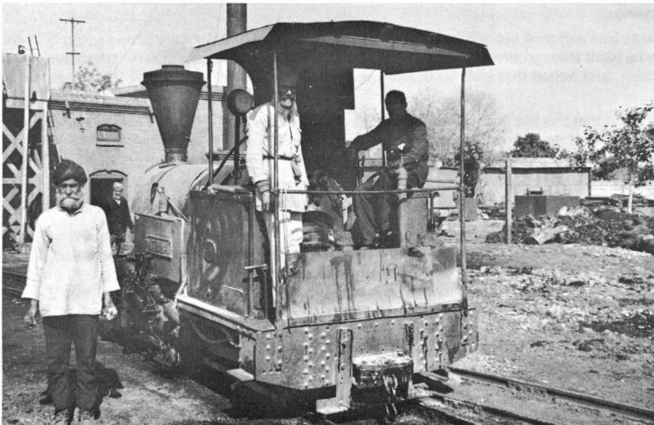
Member Mike Satow's latest find is a pair of Dick Kerr 0-4-2 inverted saddle tanks, probably the last surviving examples of locos fitted with Morton's valve gear. They are employed on the 2'6" gauge system at Dhillwah Sleeper Depot in the Punjab. Both are ex Kharachi Port Trust, MTR No. 1 dating from 1908 and its sister engine from 1910. (M.G. Satow).
