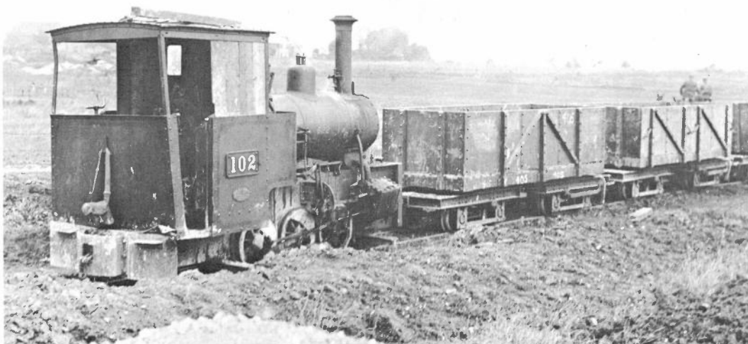
WDLR 102 in active service on a British military light railway in the Somme area. Note the two varieties of C class bogie wagon. These were an early type of wagon, produced before the decision was taken to standardise rolling stock.
