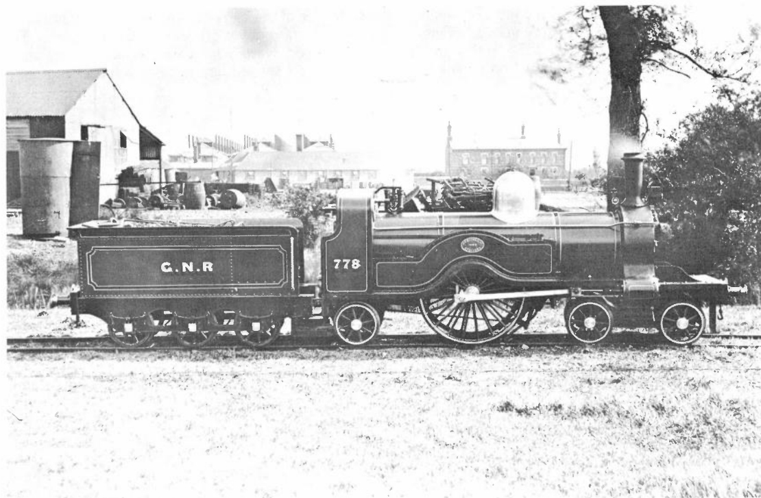
The Bagnall built Stirling single (WB 1425/93) outside Bagnall's works before delivery (Collection R.N. Redman)
