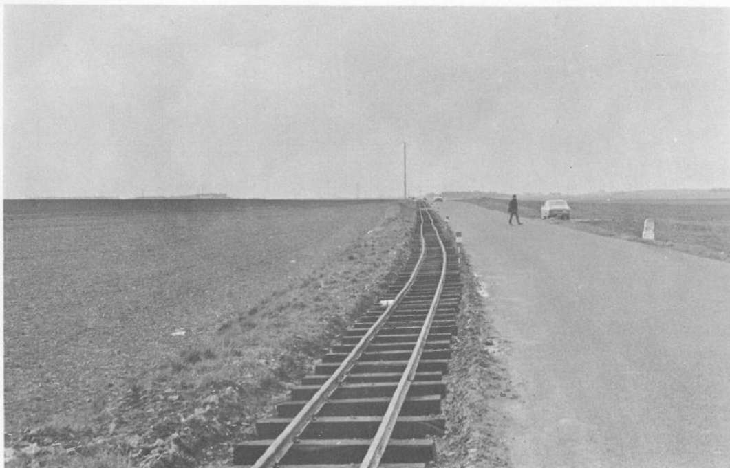
A very typical French light railway scene. The renovated section of line, showing the new sleepers and original rails before the track was ballasted and lined. March 1978. (M. Geiger)
