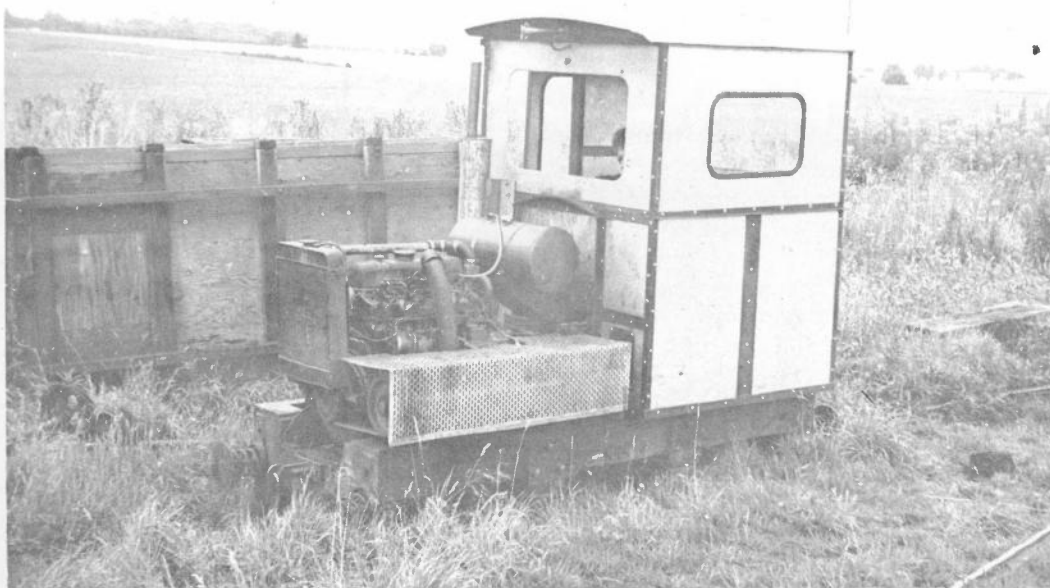
Richardson's Moss Litter Co. Ltd: The rebuilt Ruston is scarcely recognisable as a 20DL model. The perforated guard on the footplate covers the layshaft.
