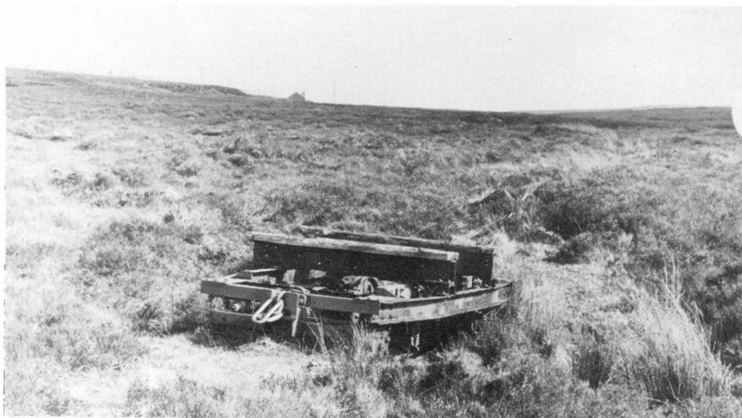
The overgrown route of the Stornoway Waterworks line looking towards the filter house. In the foreground, the Motor Rail frame. The engine bearers have been fitted with timber baulks to carry a load. (Ian B. Jolly)
